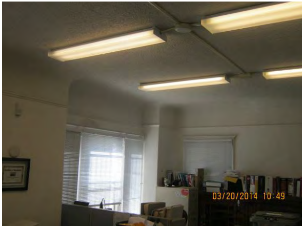
Interior view 5203 Dover Street building
