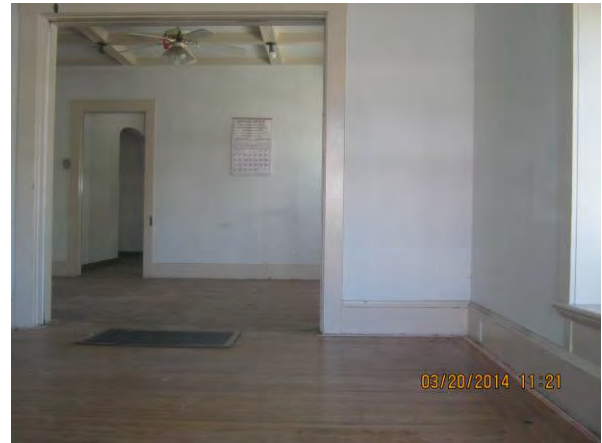
View inside of the 707 53 rd Street building
