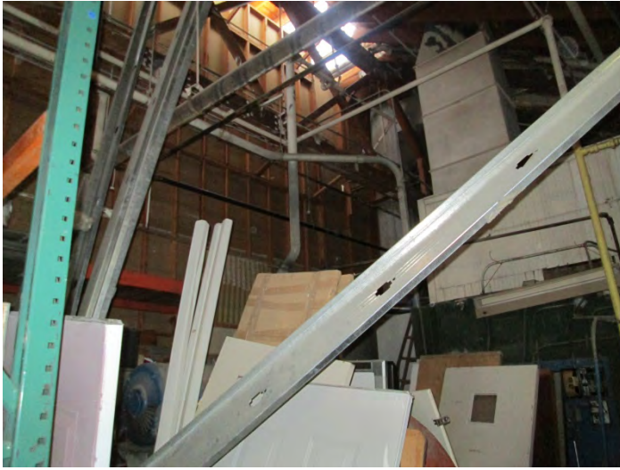
17. Additional view of the maintenance/storage room
