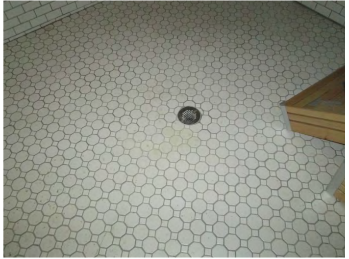
10. View of a shower floor drain
