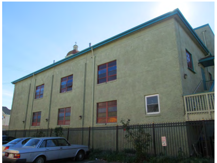
28. View of the south adjacent property (Saint John's Missionary Baptist Church)
