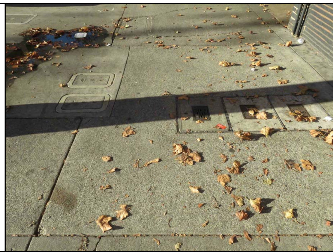
2. INTERNATIONAL BLVD. SIDEWALK LOOKING WEST
