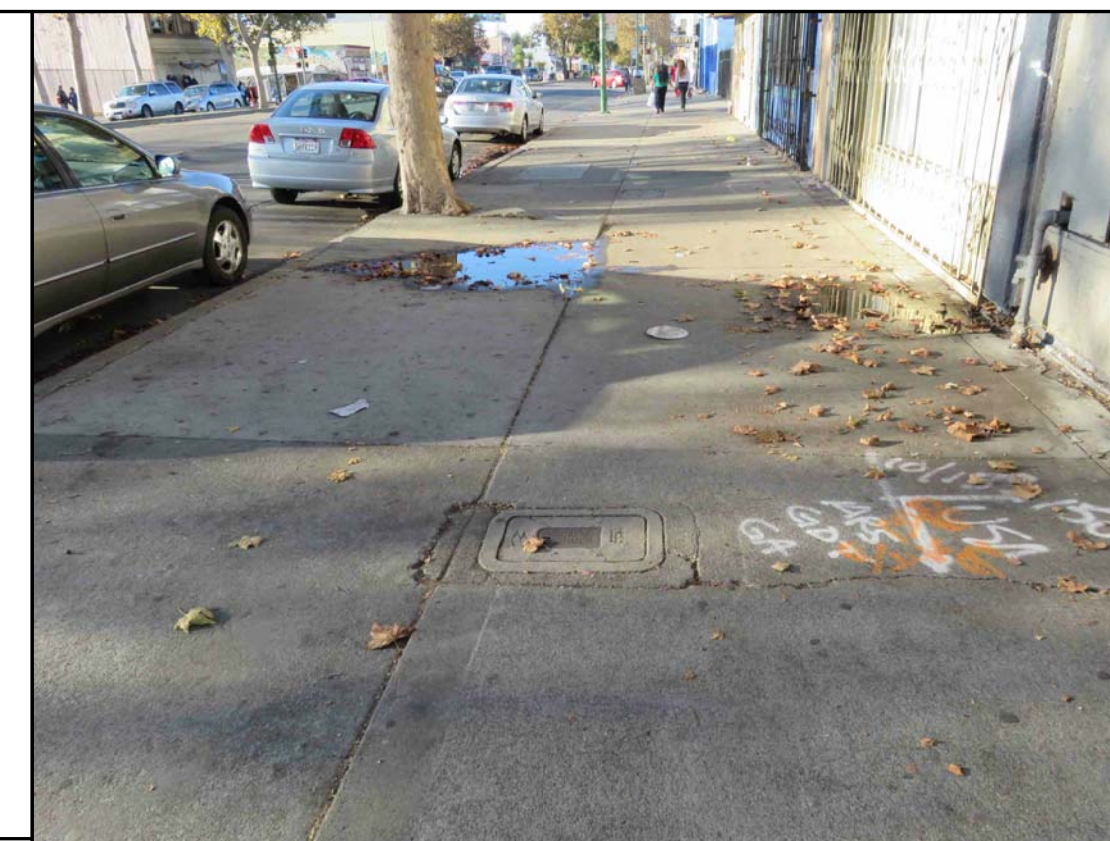
3. INTERNATIONAL BLVD. SIDEWALK LOOKING WEST
