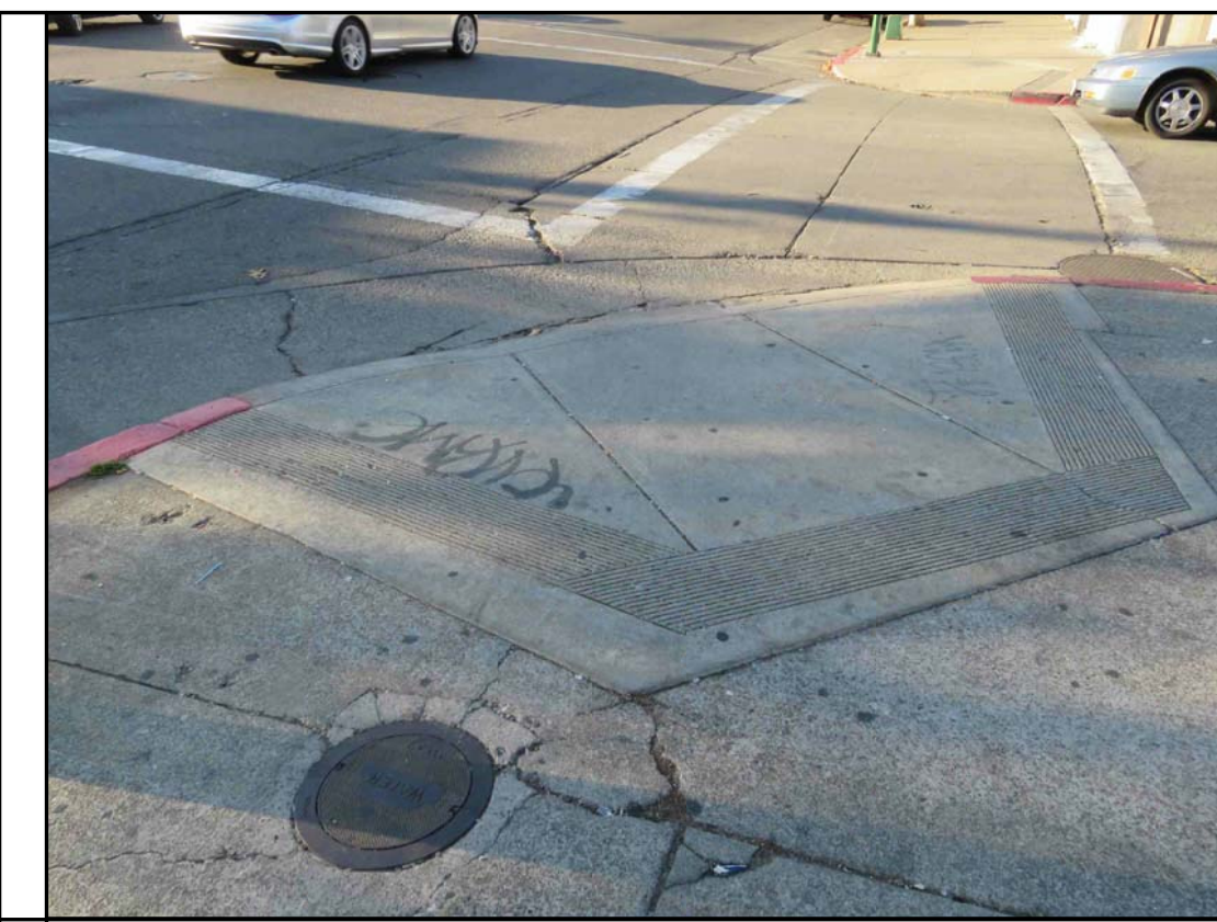
4. INTERNATIONAL BLVD. AND 94TH AVE. AT SOUTH - WEST CORNER
