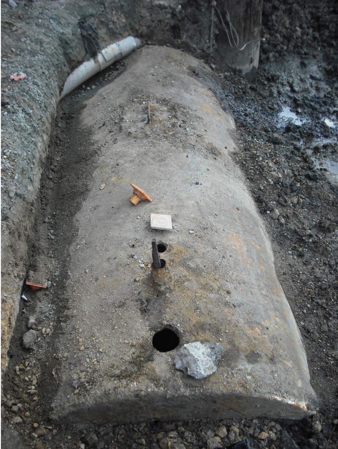
UST prior to removal
