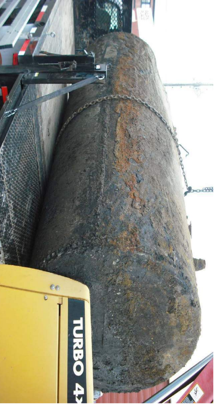
UST following removal
