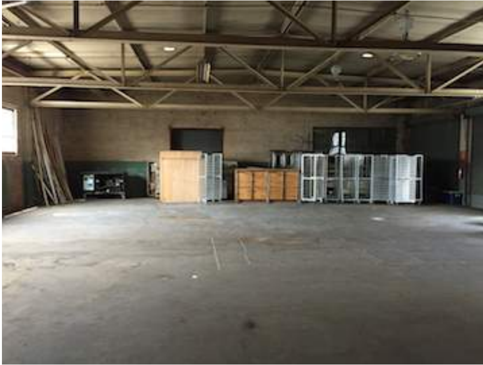
Photograph 13 – Warehouse of main building.
