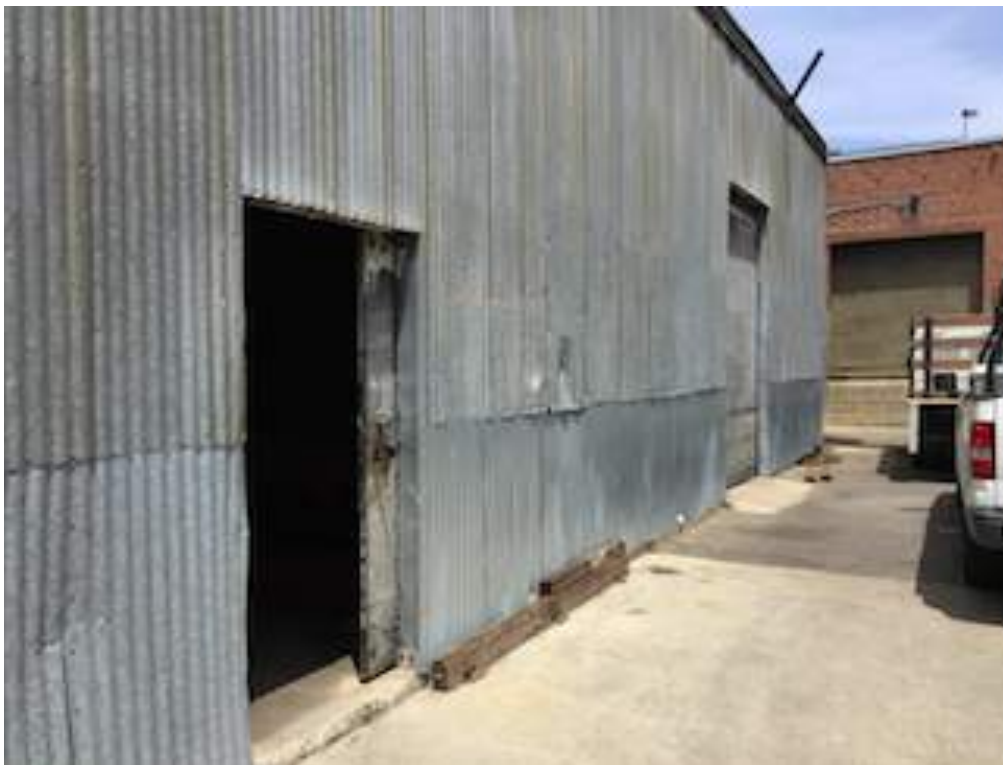
Photograph 6 – Corrugated metal maintenance shed in central portion of Property.
