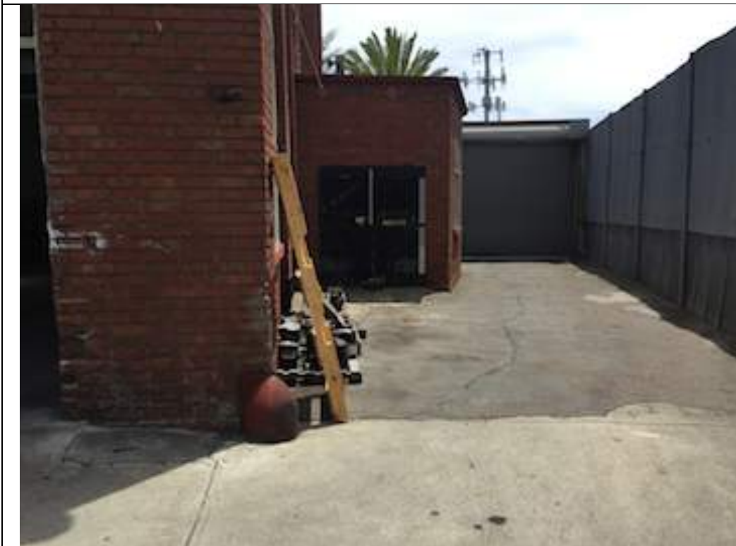
Photograph 16 – Adjacent to the wall on the left is the former pump and in the center is the former location of the closed UST.
