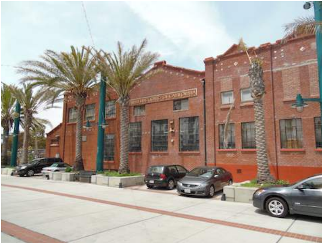
Photograph 2 - Southern wall of Property building.
