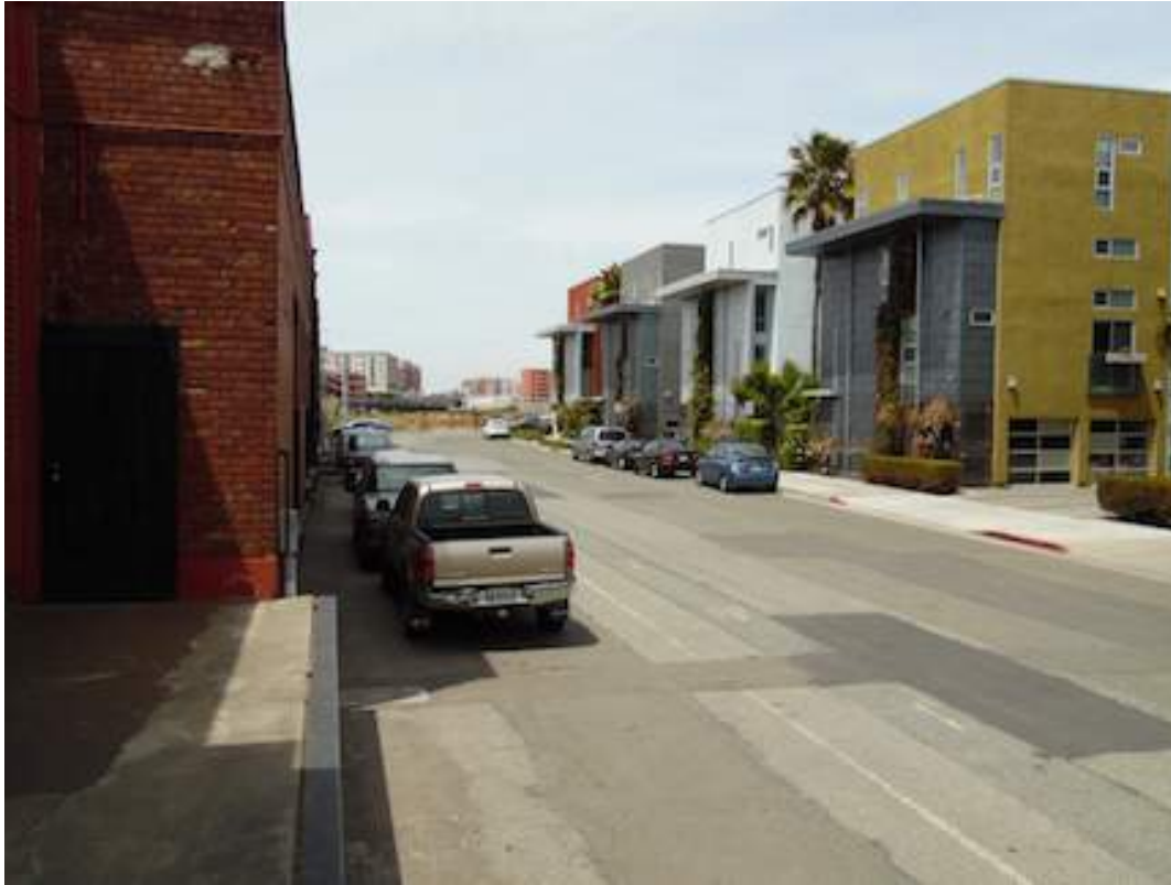
Photograph 3 – Halleck Street looking north, loading dock for Property building is on left.
