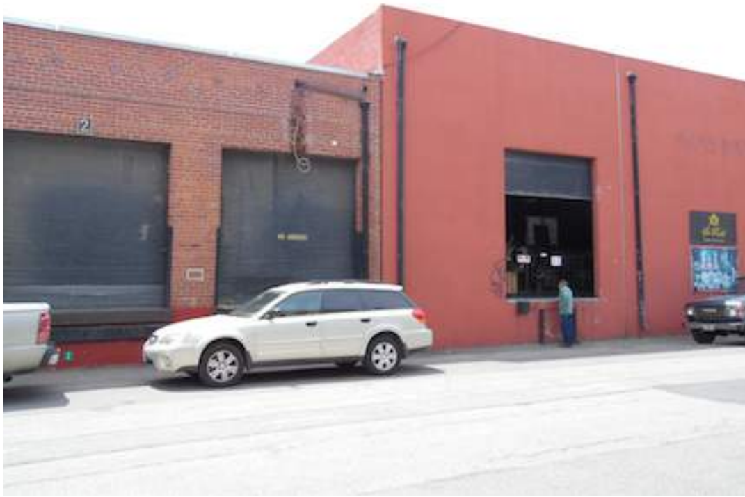
Photograph 5 – Property boundary with site to the north.
