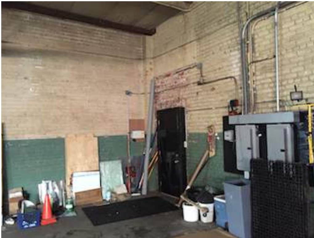
Photograph 14 – Northeast corner of main building with 5-gallon buckets of cleaners.
