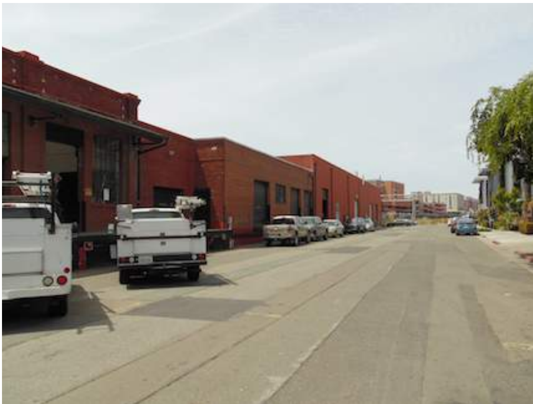
Photograph 4 – Looking north on Halleck Street at east side of Property building.
