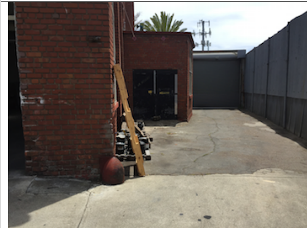
Photograph 16 – Adjacent to the wall on the left is the former pump and in the center is the former location of the closed UST.
