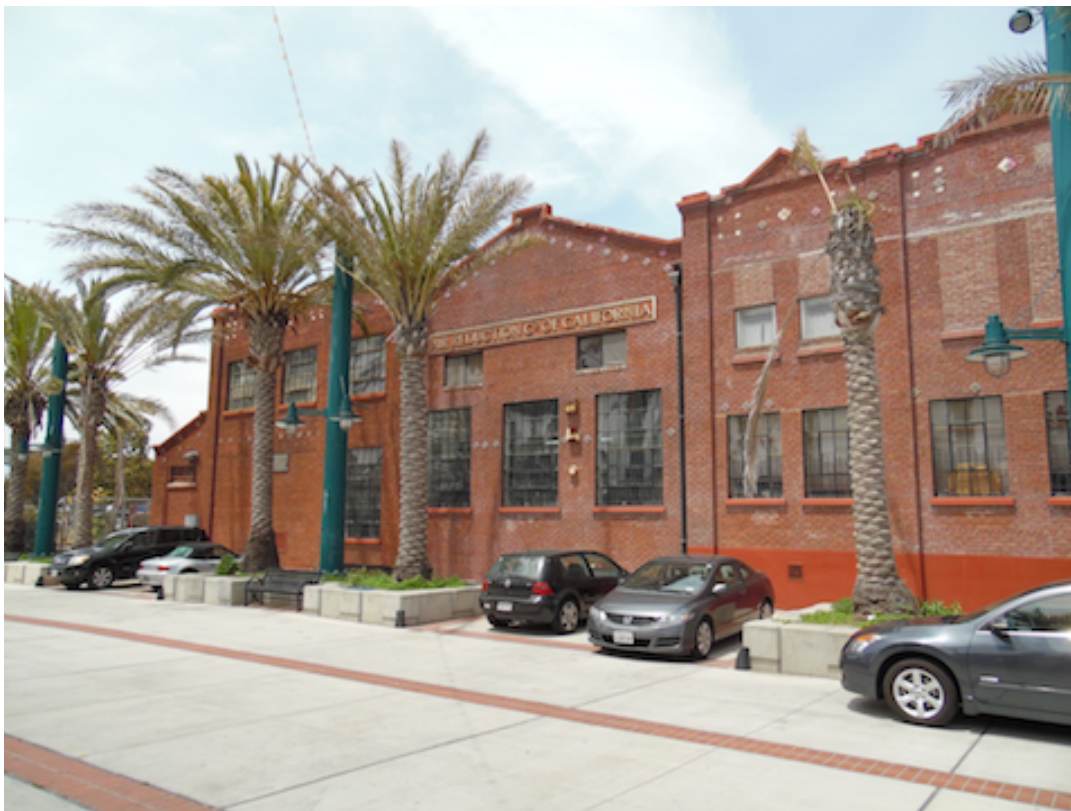
Photograph 2 - Southern wall of Property building.
