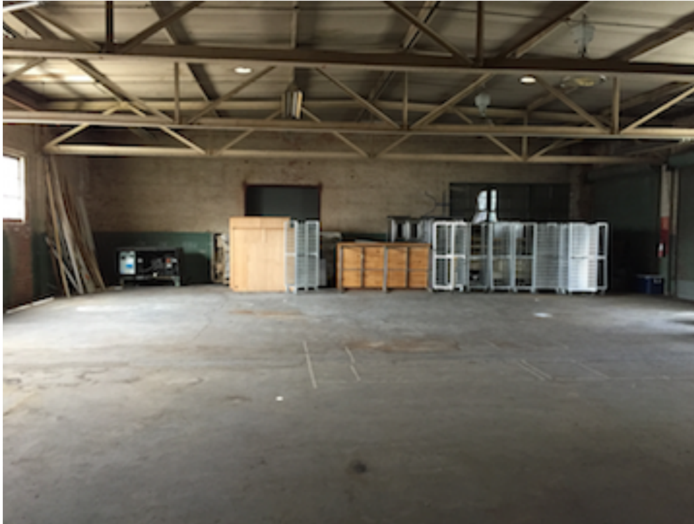
Photograph 13 – Warehouse of main building.
