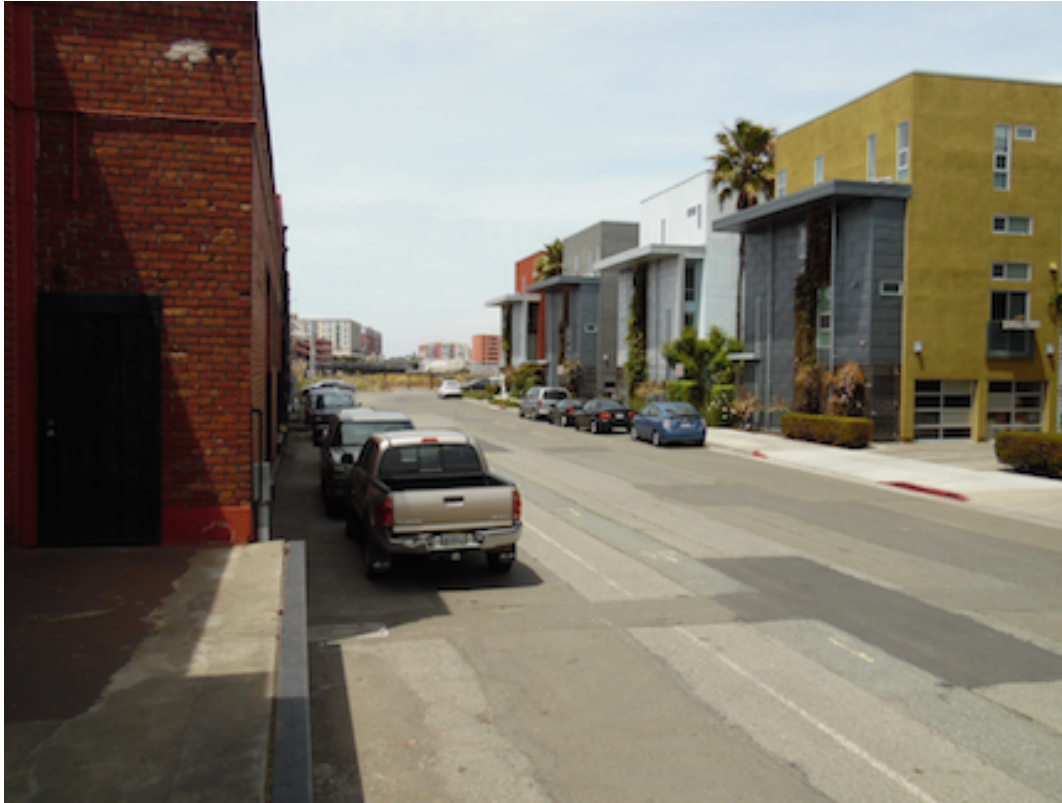
Photograph 3 – Halleck Street looking north, loading dock for Property building is on left.
