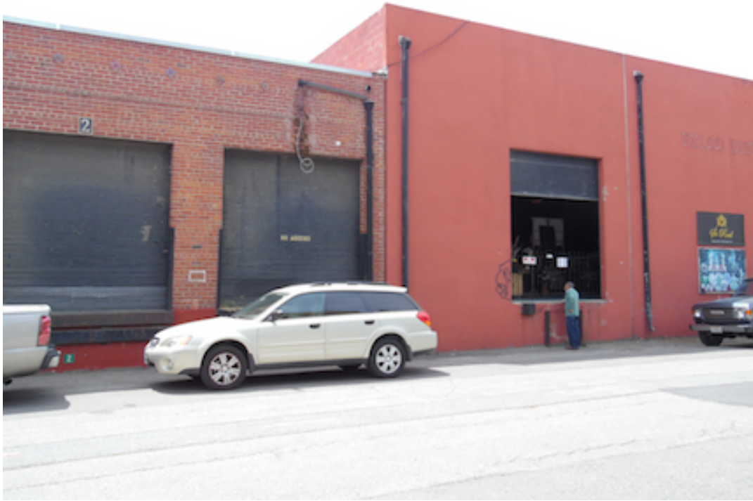
Photograph 5 – Property boundary with site to the north.
