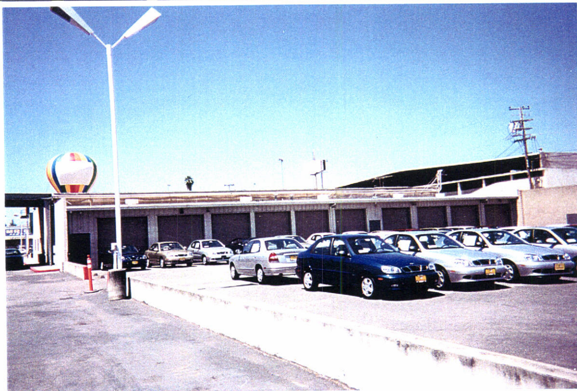
2. Maintenance shop for Lloyd Wise at 1424 105 th Avenue.
