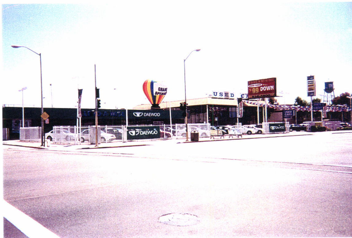
1. Automobile dealership at 10500 - 10550 East 14 th Street (view across East 14 th Street).
