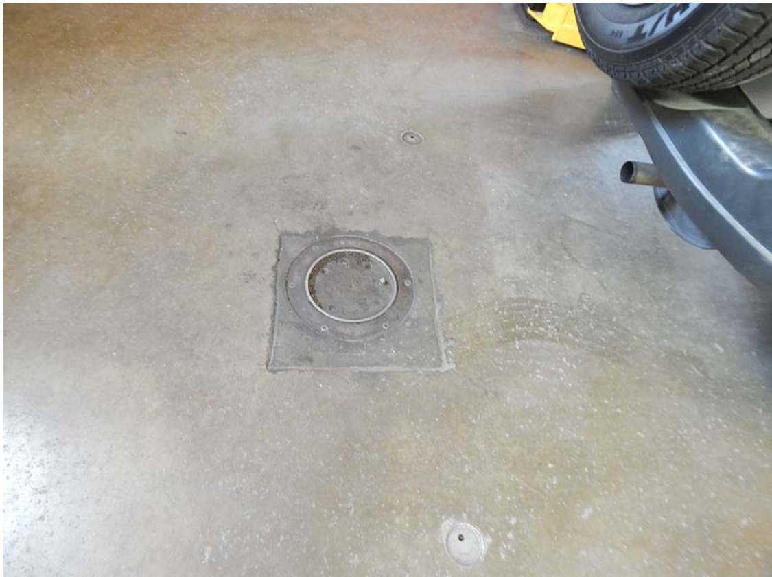
Photograph 6 - View of the disused in ground lift at 1814 Everett Street
