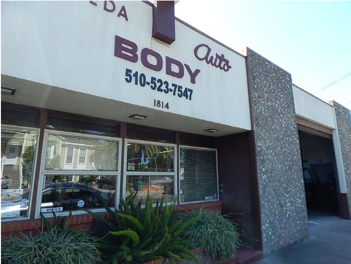
Photograph 1 - View of the 1814 Everett Street building - Alameda Auto Body
