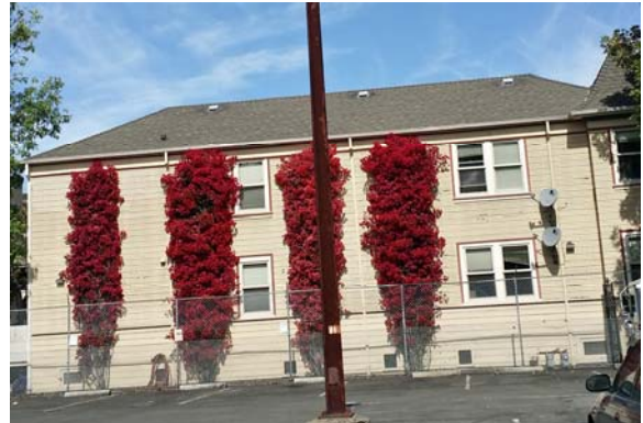
10. View west at the western adjacent property.
