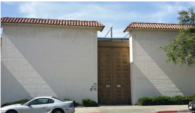
11. View south across 21 st Street at the southern adjacent property.
