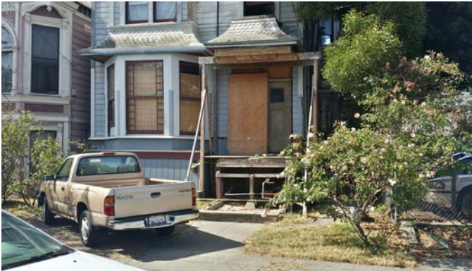
9. View south at the eastern adjacent property.
