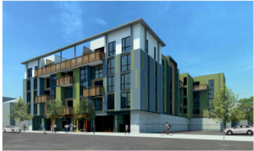
11 FRONT ELEVATION AT 21ST ST. - LOOKING NORTH
