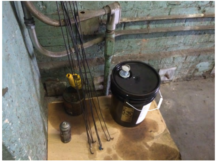
30. A five-gallon barrel labelled "CO-400 High Temperature Chain Oil" located near the furnace area, with staining
