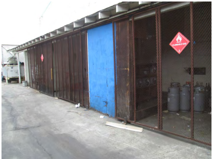
4. Hazardous substances storage area southeast of the subject property building
