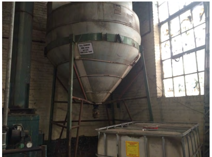
12. Additional hazardous materials storage located in east side of warehouse
