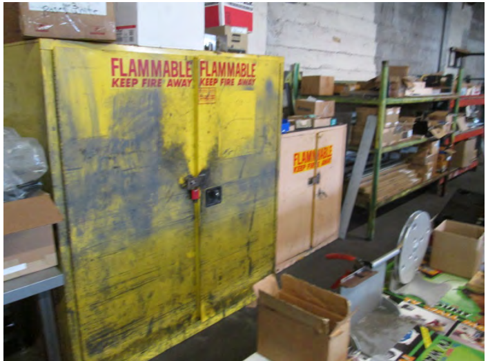
16. Storage closets located in the northwest section of warehouse; no hazardous substances found in the closets
