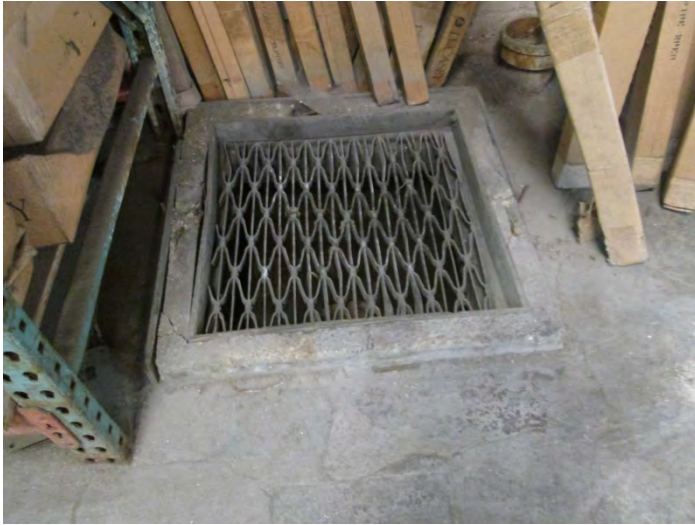
9. Floor drain located in the east side of the warehouse
