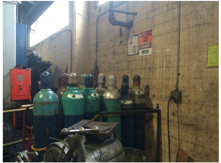
26. Compressed gas cylinders of Carbon Dioxide and Argon, located in the west section of the warehouse
