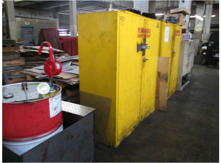
18. Hazardous substances storage containment located in the southwest section of the warehouse
