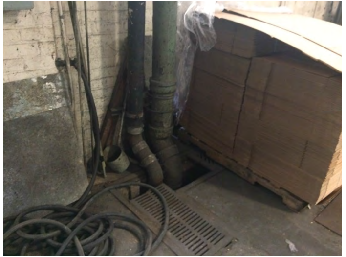
10. Floor drain located in east side of warehouse
