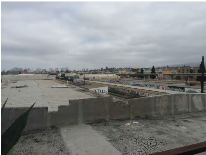
35. View of roof access located on the fourth level
