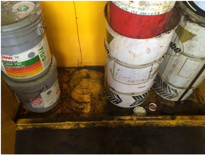
21. View of the lower area of hazardous substances closet #1
