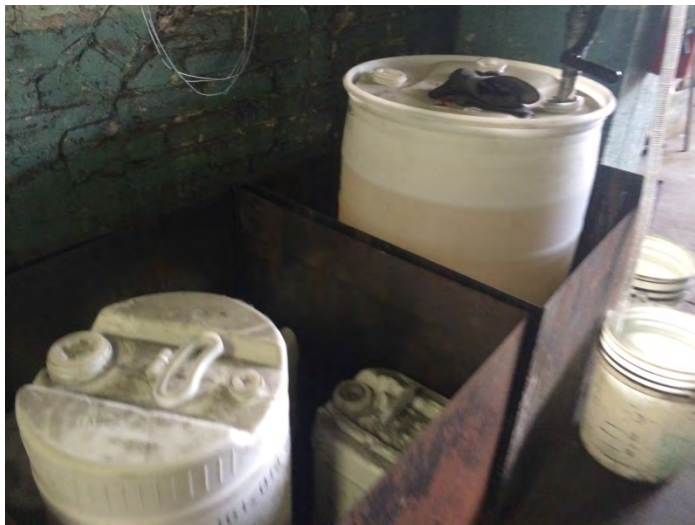
31. Unidentified substance containers with secondary containment, located near the furnace
