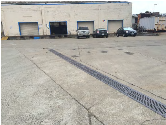
39. View of a storm drain and patched areas, east side of subject property
