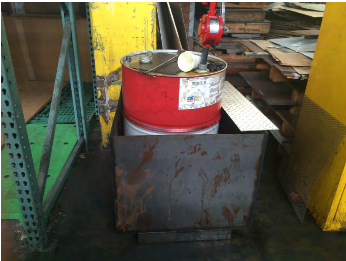
19. A 55-gallon oil tank labeled "Teresstic 68" with secondary containment found in the southwest section of the warehouse
