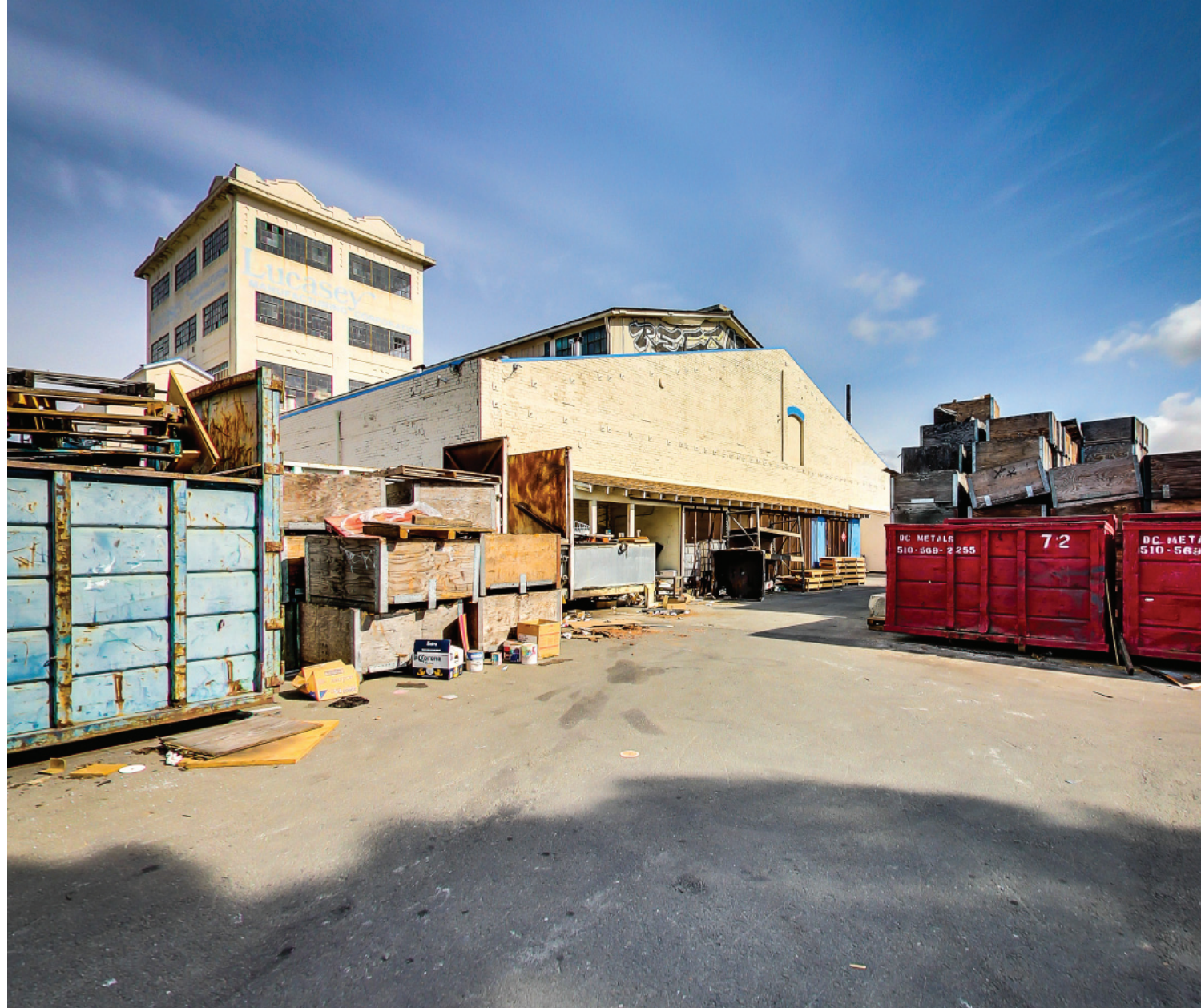
Existing Site Photo
