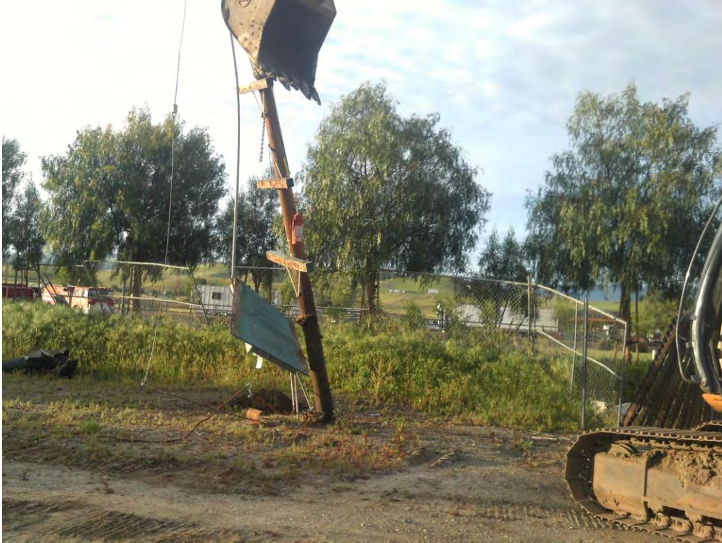
Photograph 1: Facing south at the power pole removal prior to excavation activities.
