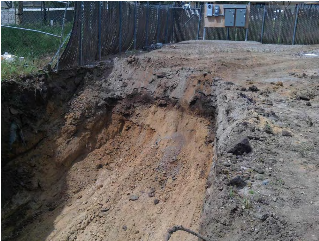
Photograph 4: Final west extent of excavation.
