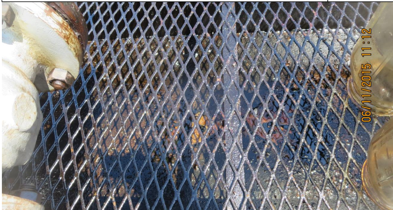
DESCRIPTION: VIEW OF INSIDE OF FUELING SPILL CATCHING BASIN
