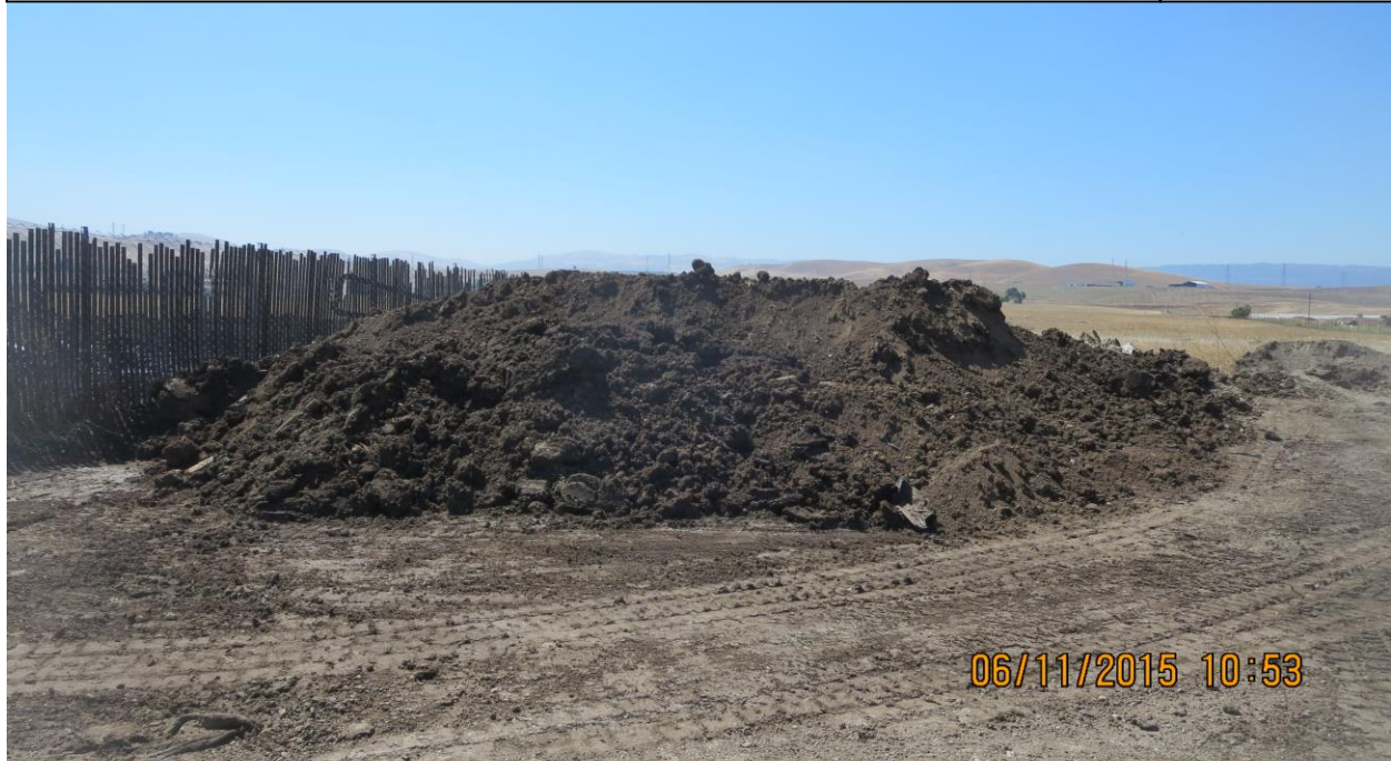
DESCRIPTION: PILE OF SOIL FROM SITE'S EXCAVATION Photo # 2 of 26
