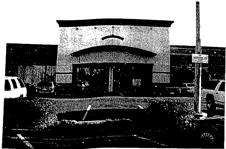
2. A view of the subject property from Chestnut Street.
