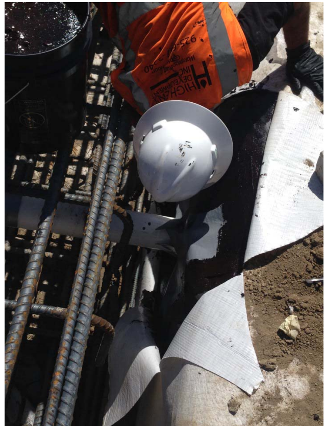
Photo 1. A plumbing penetration of the vapor barrier at the northeastern elevator pit footing of Building A. Photograph taken on April 20, 2017.
