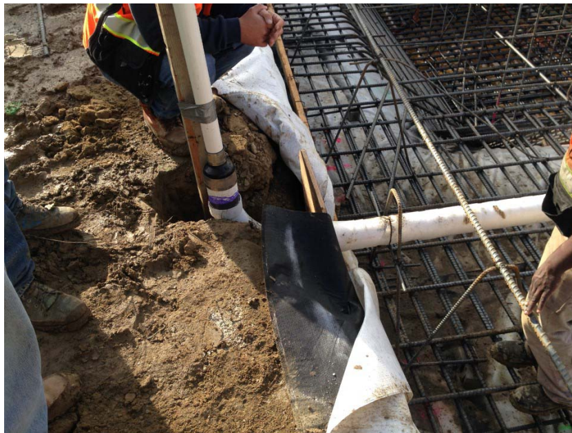
Photo 1. A plumbing penetration of the vapor barrier at the northeastern elevator pit footing of Building A. Photograph taken on April 20, 2017.
