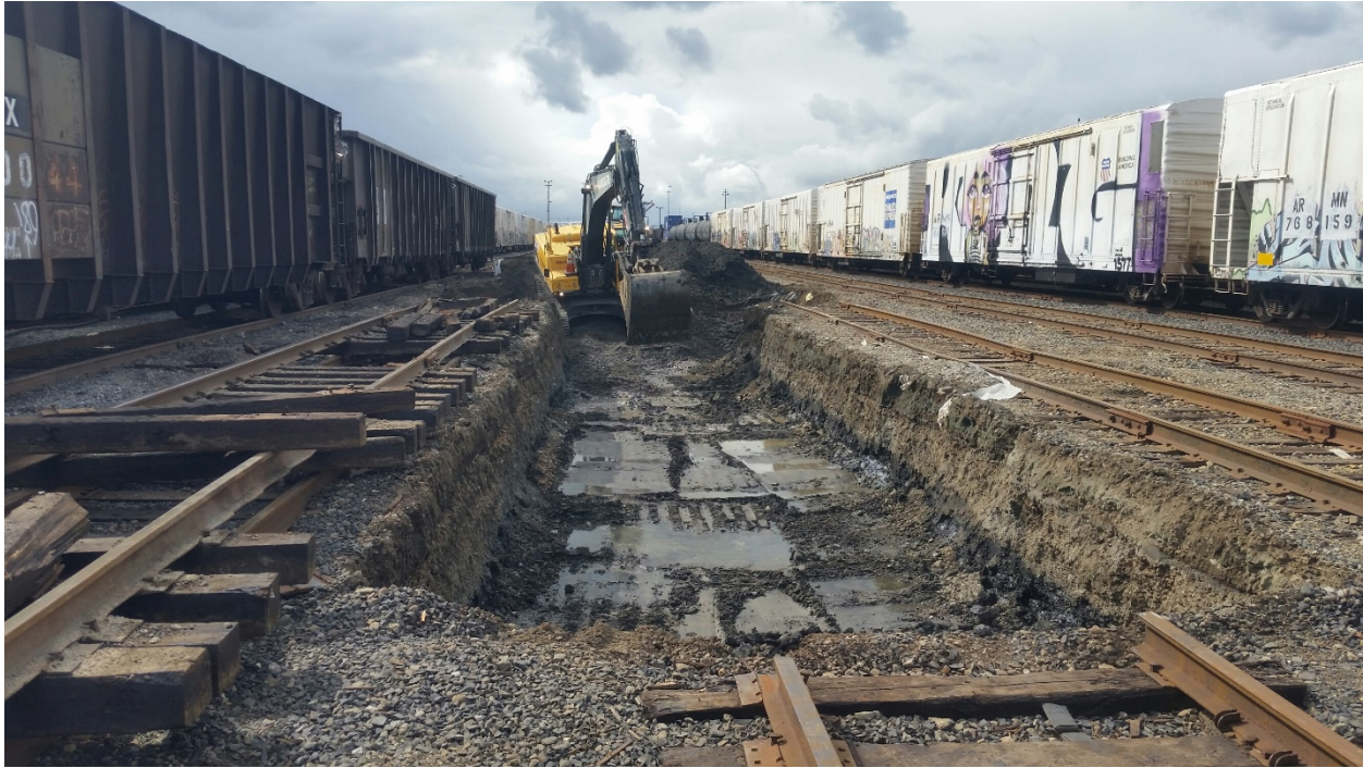
04.07.2015 Excavation view with water in the bottom of the excavation.
