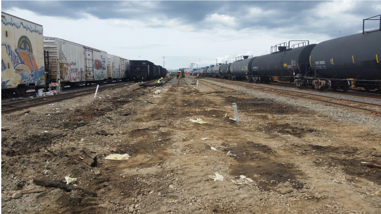
04.06.2015 Tracks 57, 58, and 59 rail removal complete.
