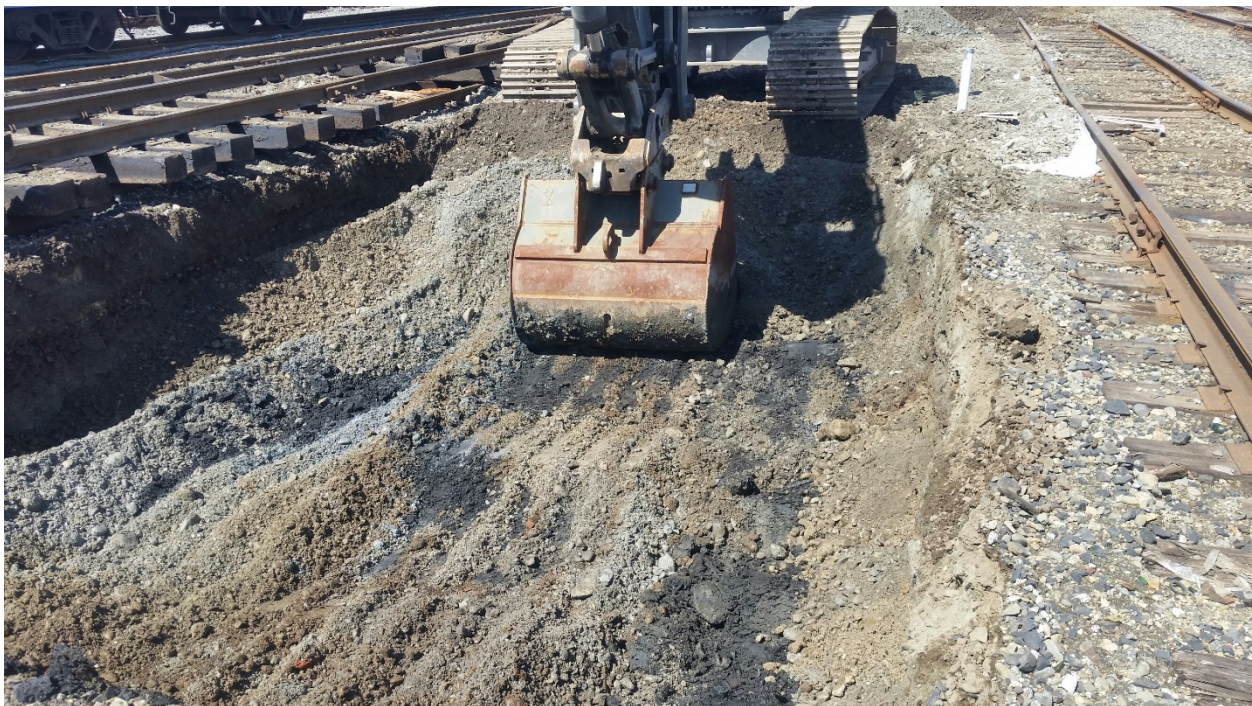
04.07.2015 Excavation activities, excavation started at the northern end.
