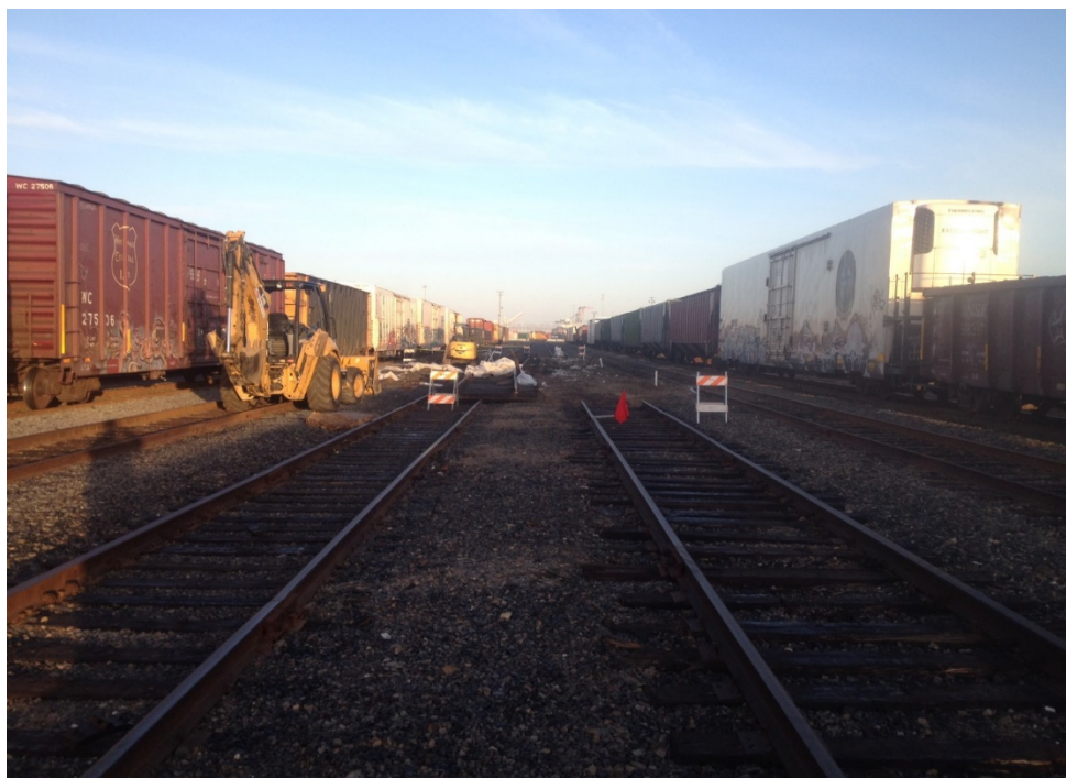
03.28.2015 Track 58 rail removal activities.
