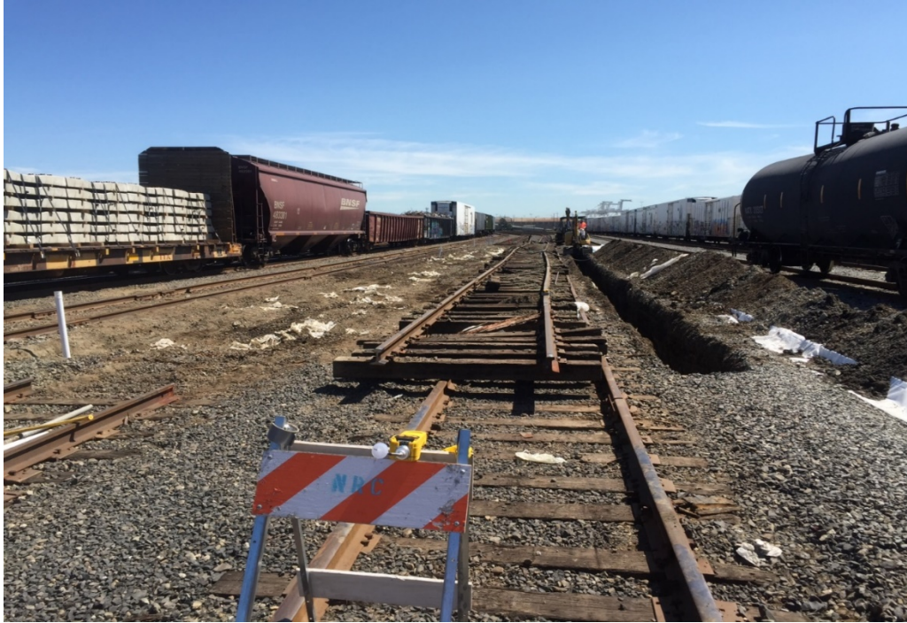
03.28.2015 Track 58 rail removal complete and Trench 3 excavation is visible.
