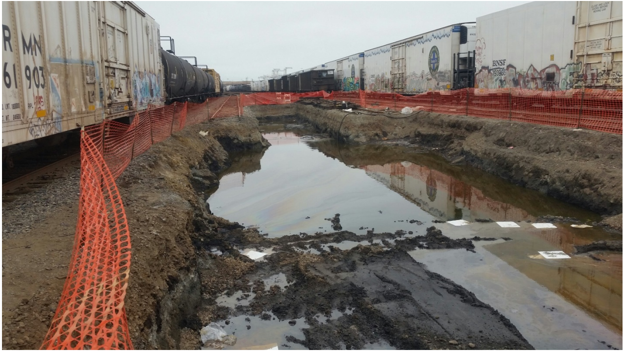
04.20.2015 Excavation view, excavation complete.
