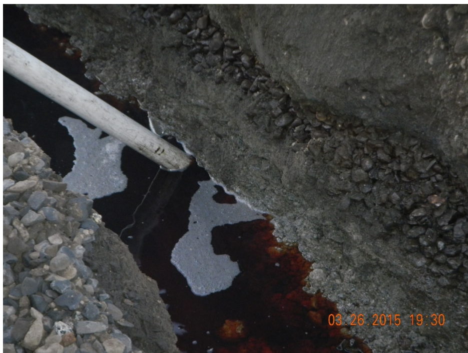
03.26.2015 Vacuum pumping begins in recovery Trench #1.
