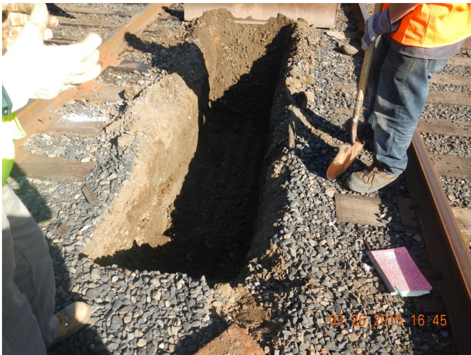
03.26.2015 Trench #1 excavation begins along west side of Track 58.
