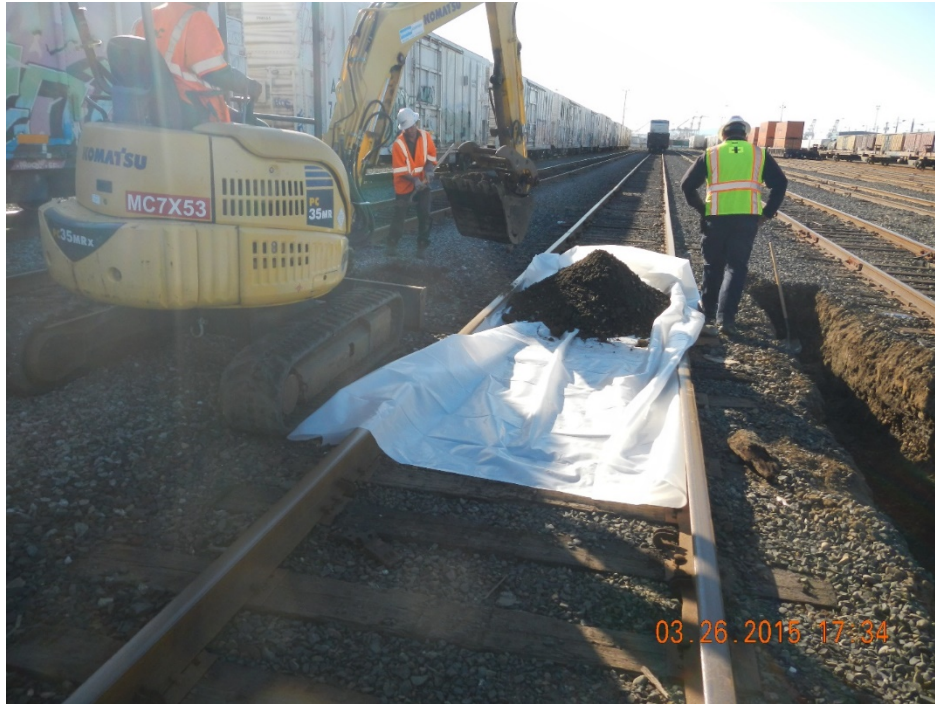
03.26.2015 Trench #1 excavation completed, Trench #2 excavation begins on opposite side of Track 58.
