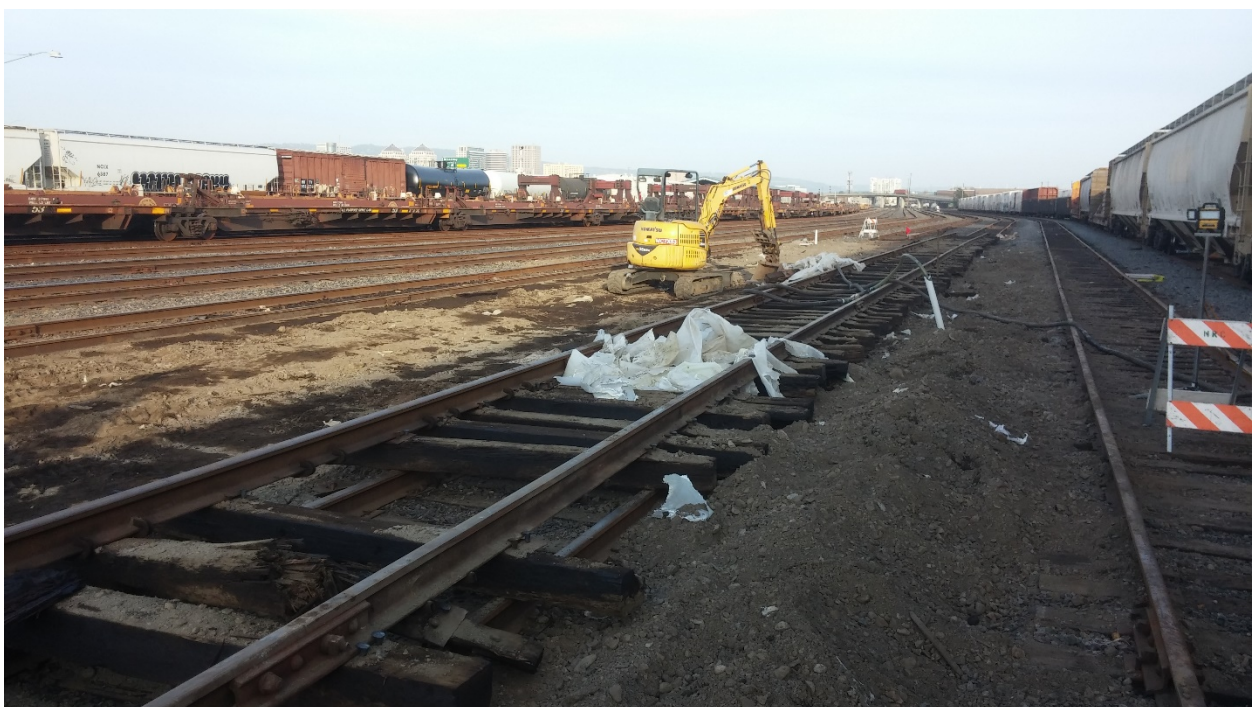
03.30.2015 Trench 3 PVC piping installation activities.
