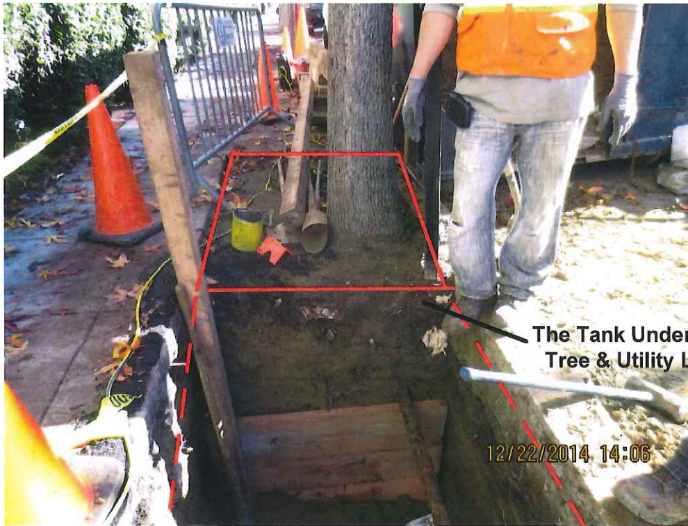
The Tank Underneath Tree & Utility Lines
