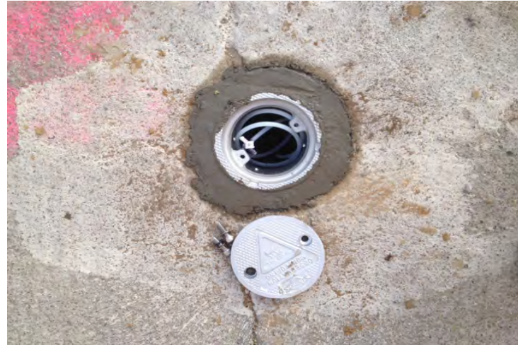
Permanent Soil Vapor Monitoring Well Completion
