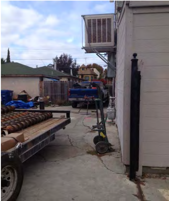
View at rear (south) of building
