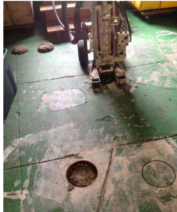
Cored slab, Indoor Limited Access Drilling
