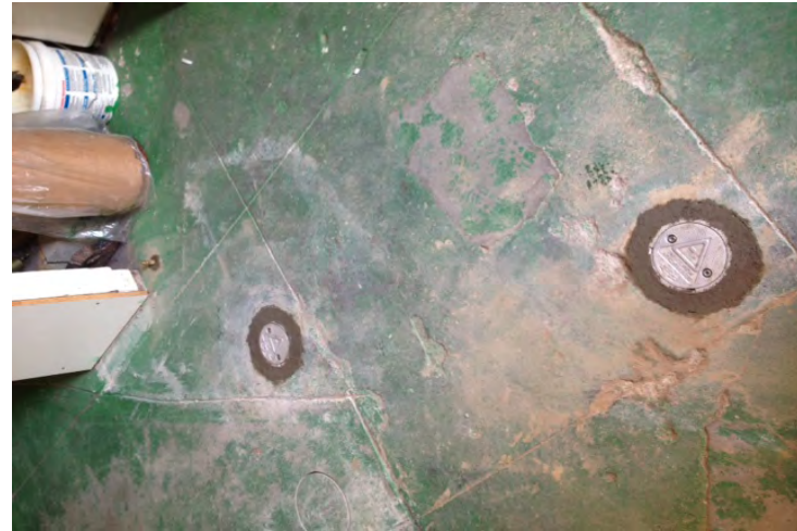
Showing indoor well completions and condition of concrete.
