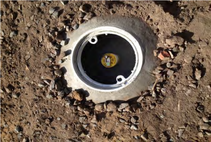
View of Monitoring Well Completion - 2 inch PVC casing.
