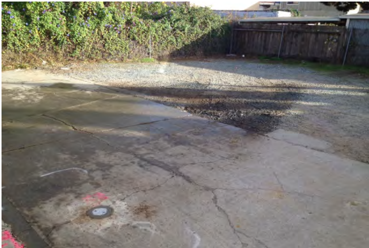
View of southern gravel parking lot and VW-3.
