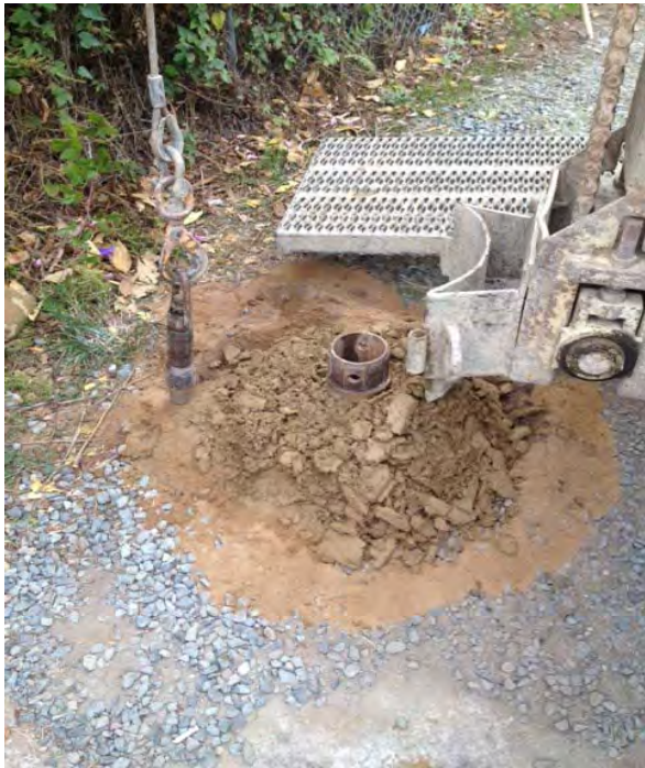
Hollow Stem Auger Drilling for Groundwater Monitoring Well
