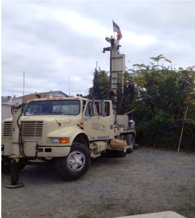
Drill Rig on Site, south of building in gravel lot.
