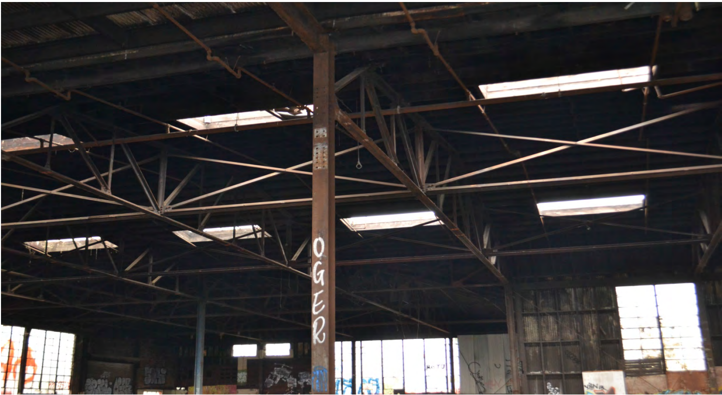
5-Ceiling of the building
