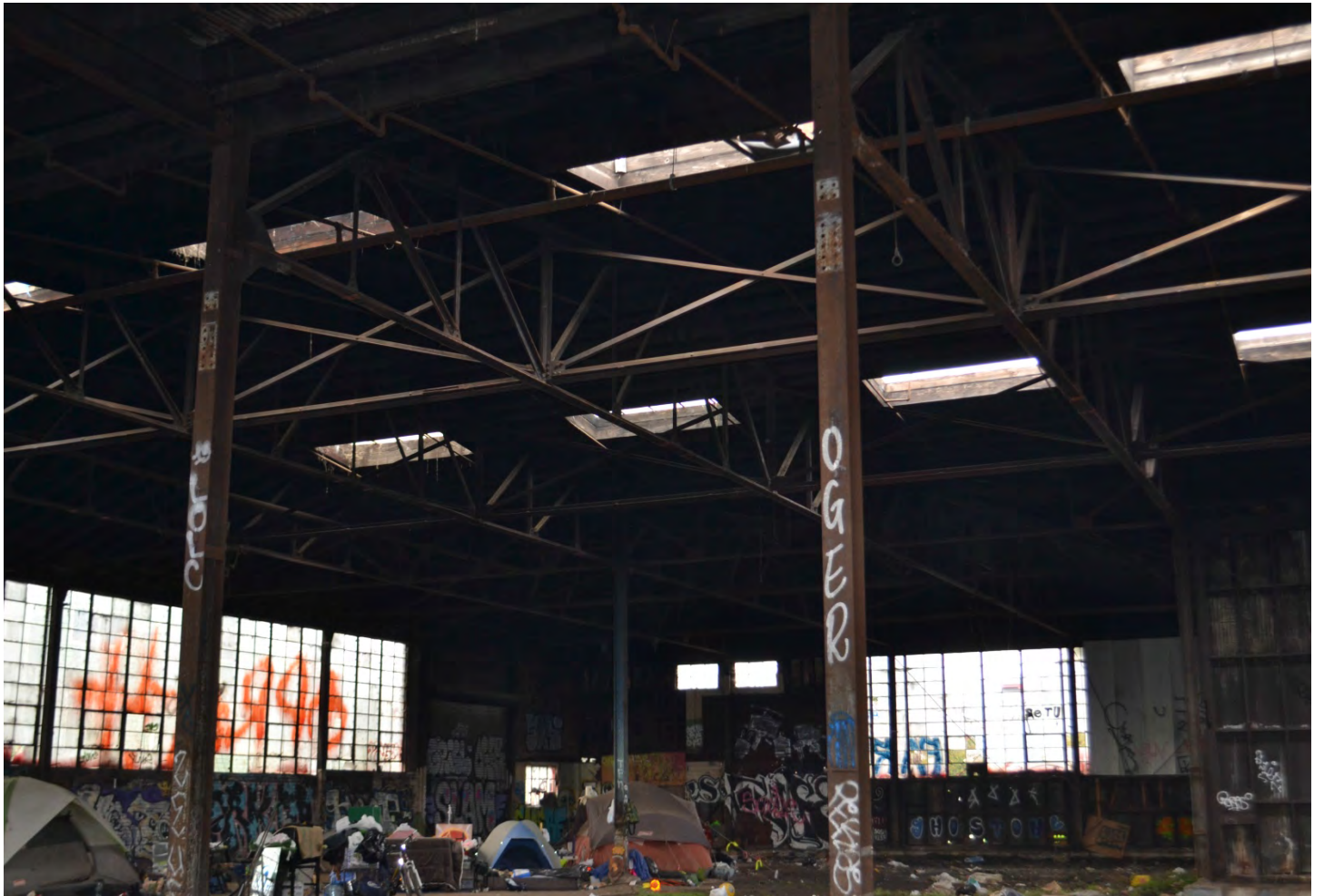
4-Interior of the Building
