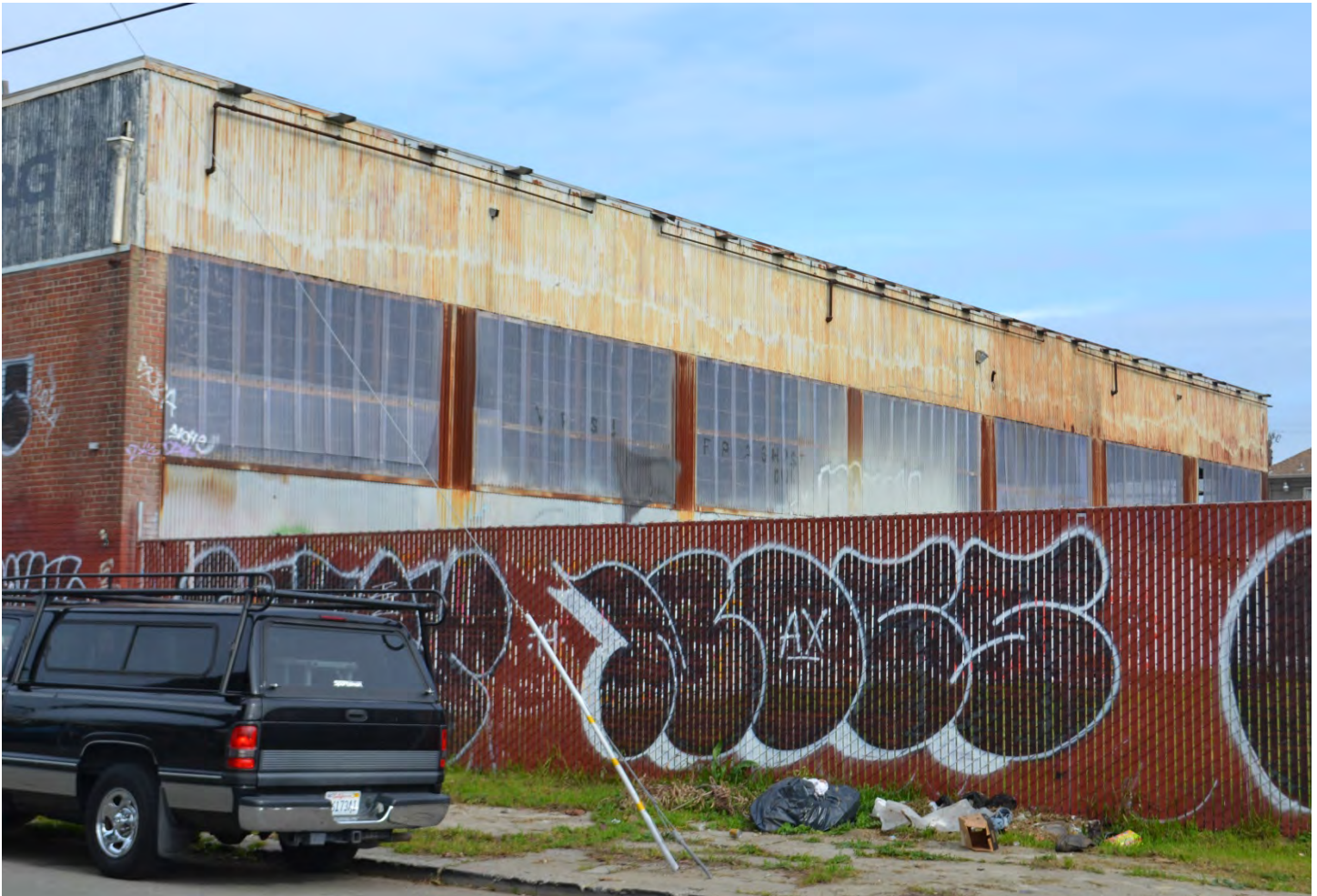
2-Southwestern side of building
