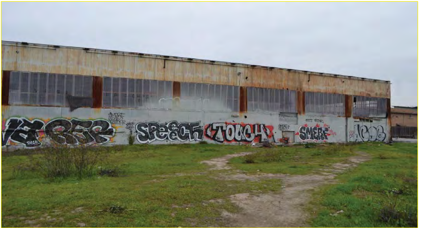
3-Southern view of Building a the Site
