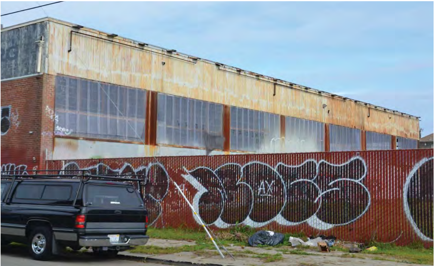
13-Southwestern side of building
