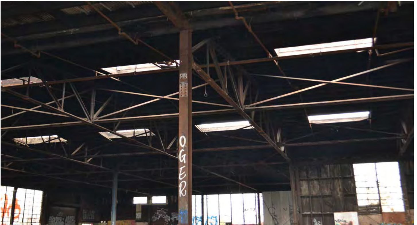
6-Cieling of building
