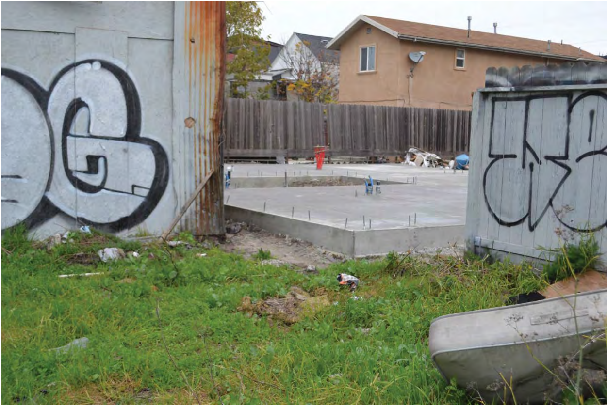
Page 2 Close up of Backyard at 2851 Helen showing Concrete building pad.
