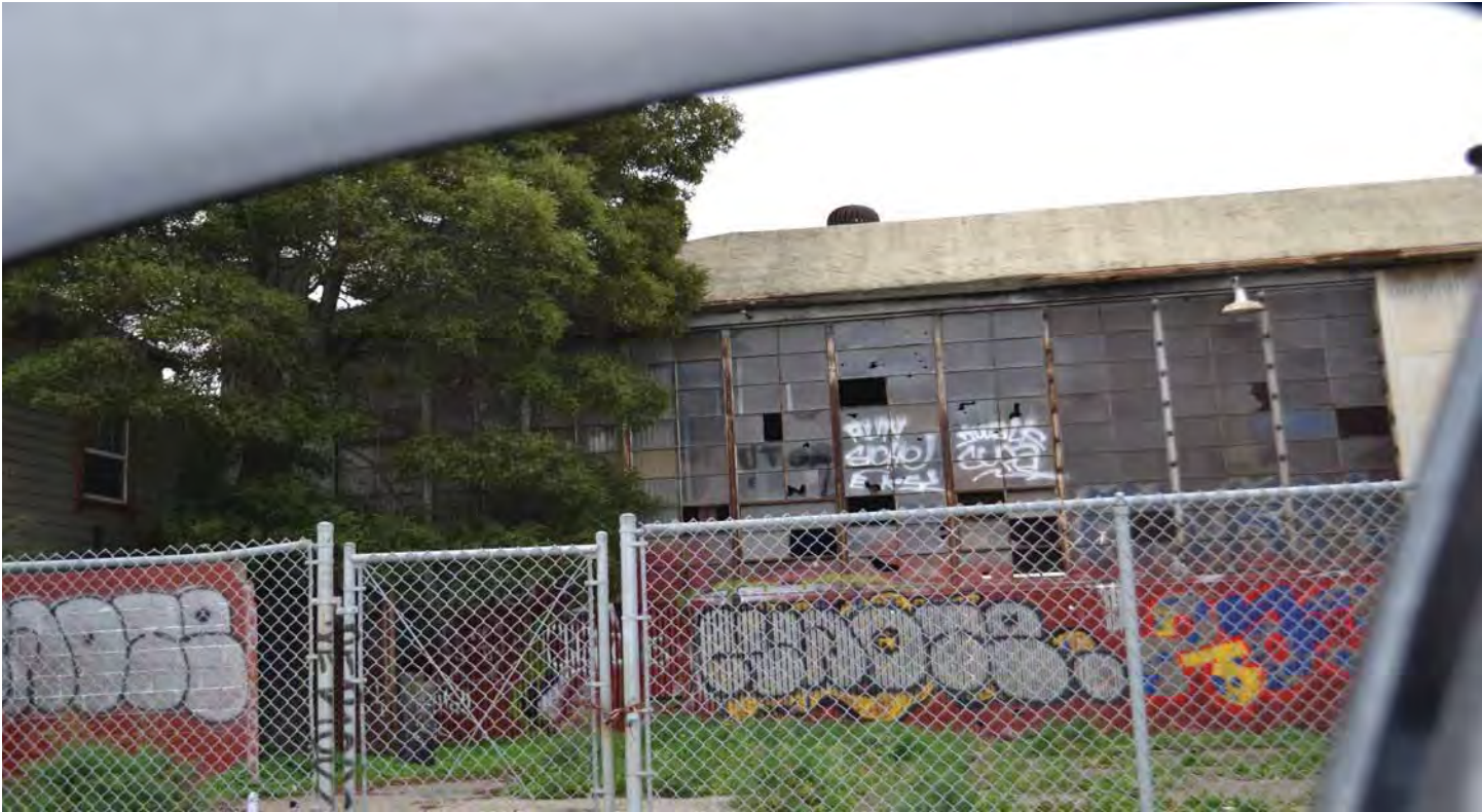
8-Northern end of building
