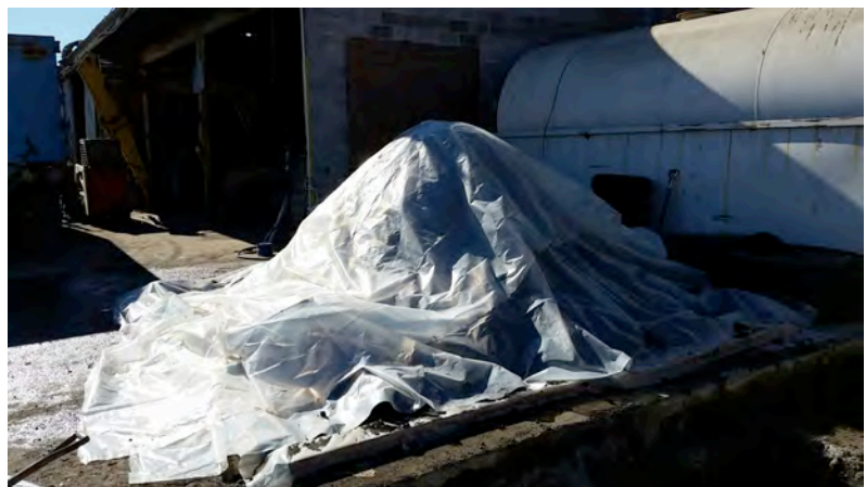
Stockpiled soil was covered with plastic sheeting following the excavation activities.
