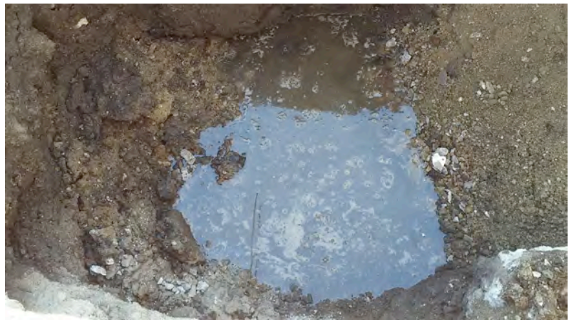
View of water in the western portion of the excavation.
