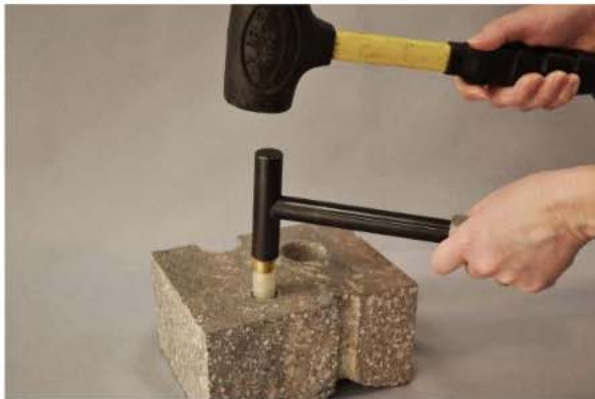
Figure 2. Installing the Vapor Pin™.
