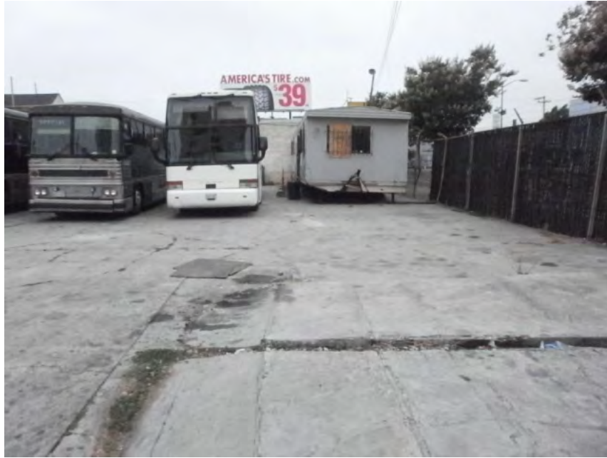
Photo 1. Portable building located on 760 22nd Street property.
