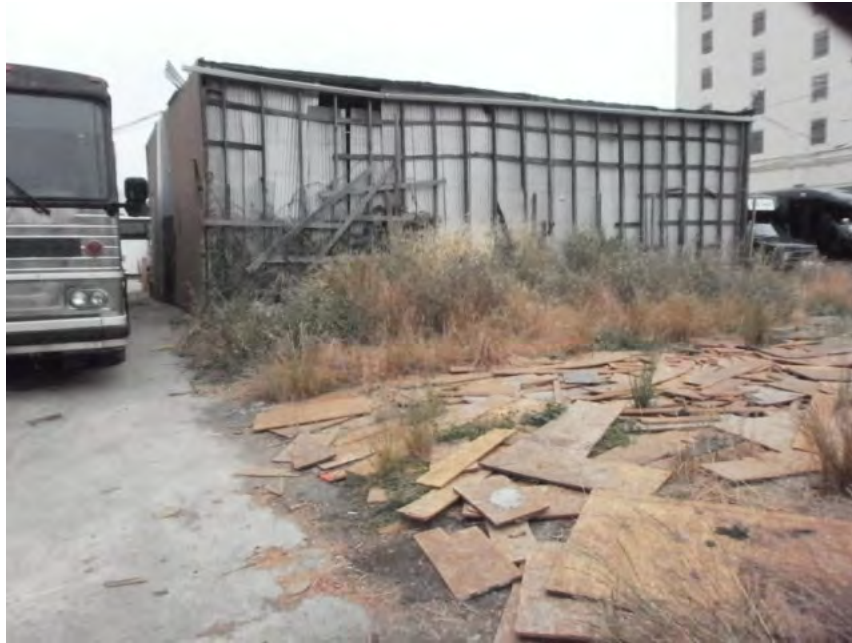
Photo 1. Metal building at 760 22nd Street and debris covering 2201 Brush Street property.
