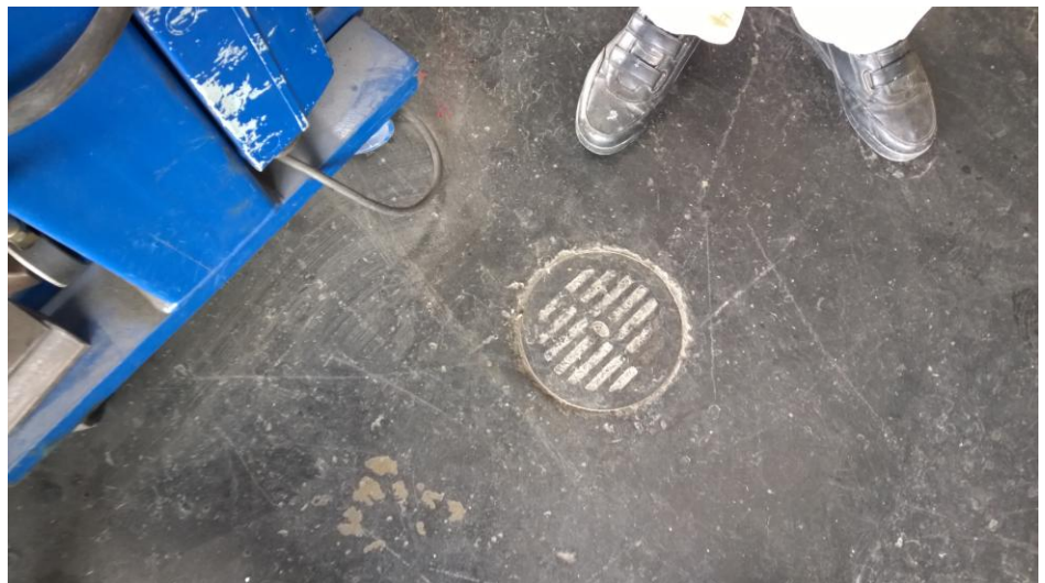
CONCRETED CLOSED DRAIN
