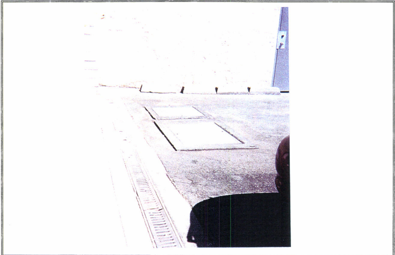
3. Oil/water separator at Lloyd Wise maintenance shop (1424 105 th Avenue).
