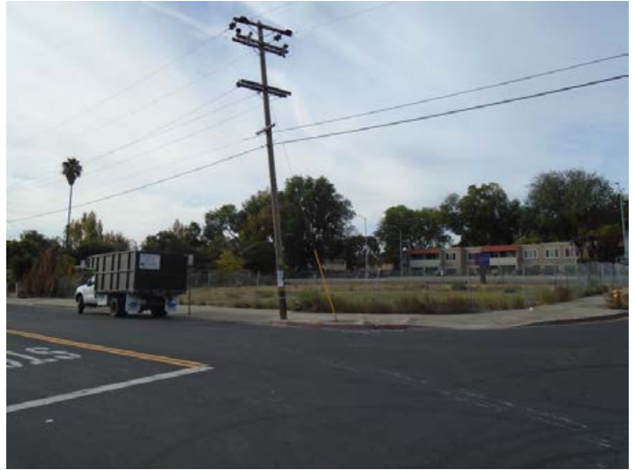
2. View of the subject property from the intersection of Loyola Avenue and Bolero Avenue, facing southeast.
