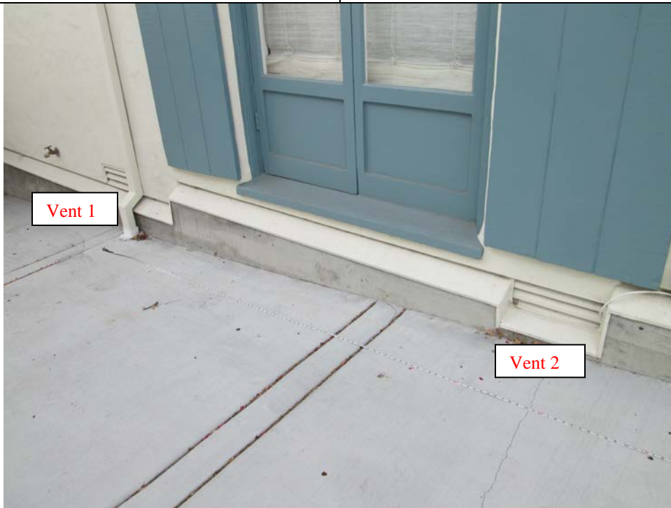
Subject: Crawl space vents on east side of residence
