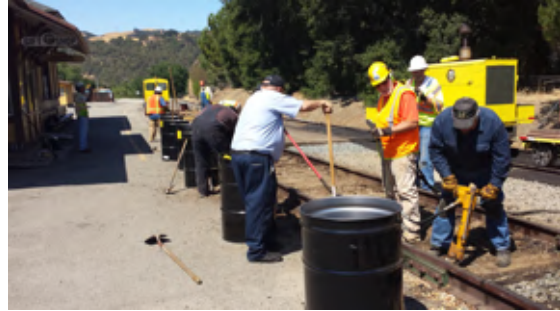
VIEW OF SOIL EXCAVATION AND REMOVAL ACTIVITIES
