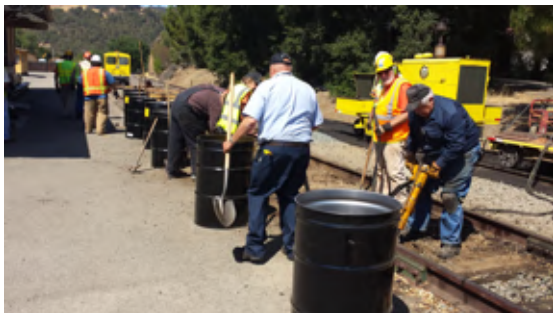
VIEW OF SOIL EXCAVATION AND REMOVAL ACTIVITIES
