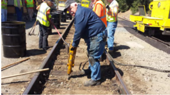
VIEW OF SOIL EXCAVATION AND REMOVAL ACTIVITIES
