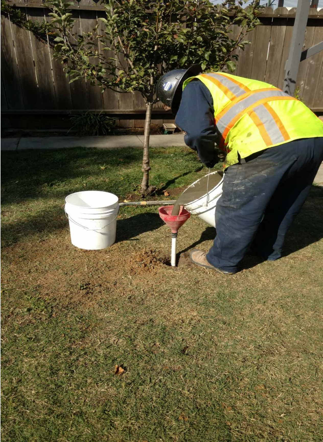
Grouting Soil Boring SB-7 Figure 7
