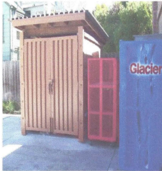
Groundwater Monitoring Well MW-3 (probably below the solid waste storage area)
