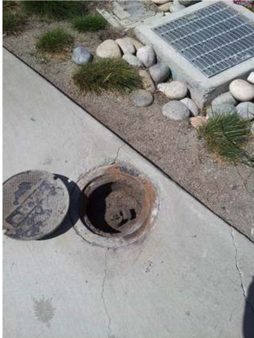
1716 Webster Street, Alameda MW-1; June 6, 2014
