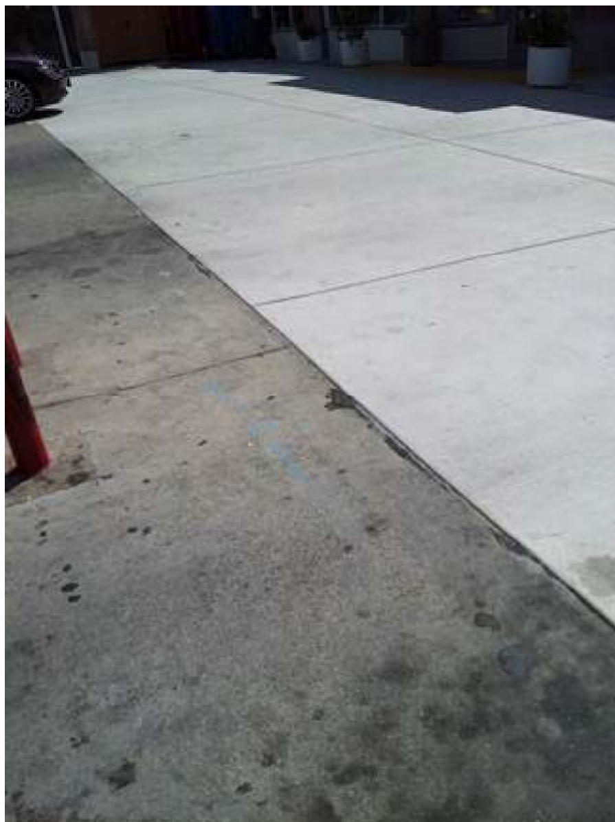
1716 Webster Street, Alameda MW-2; June 6, 2014
