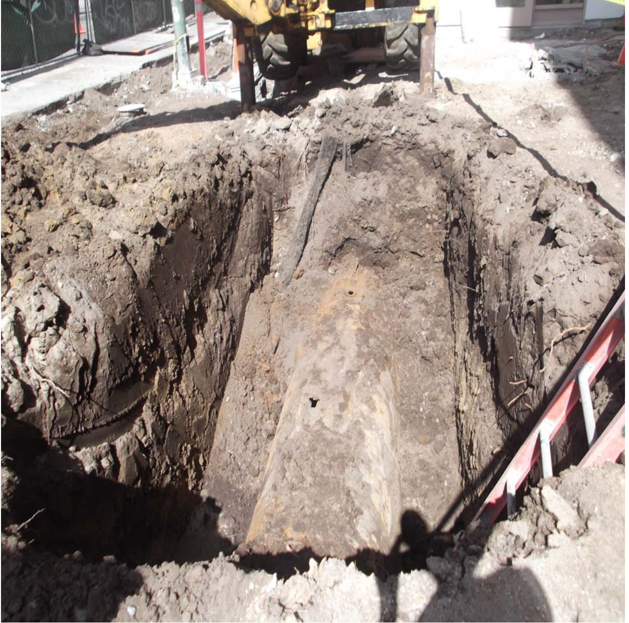
UST prior to removal
