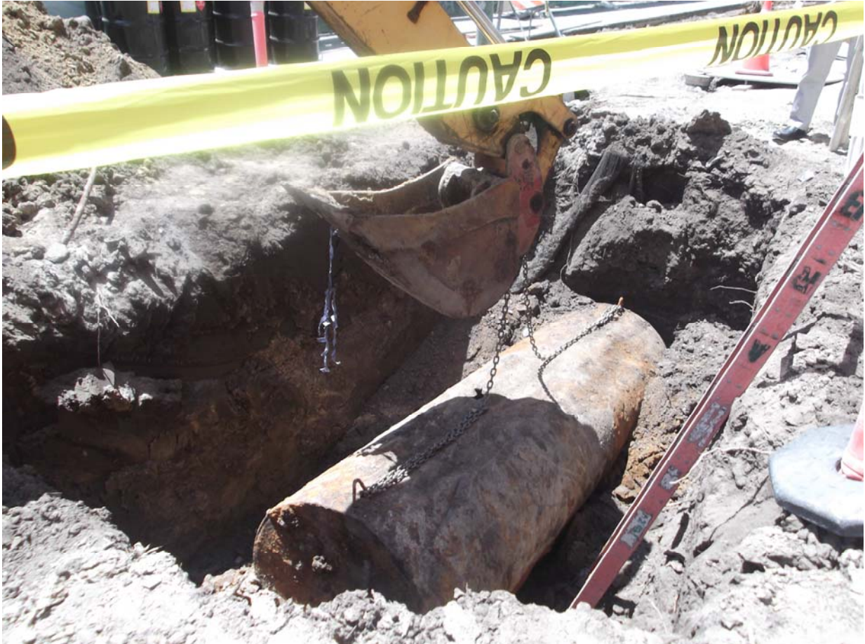
UST at the time of removal
