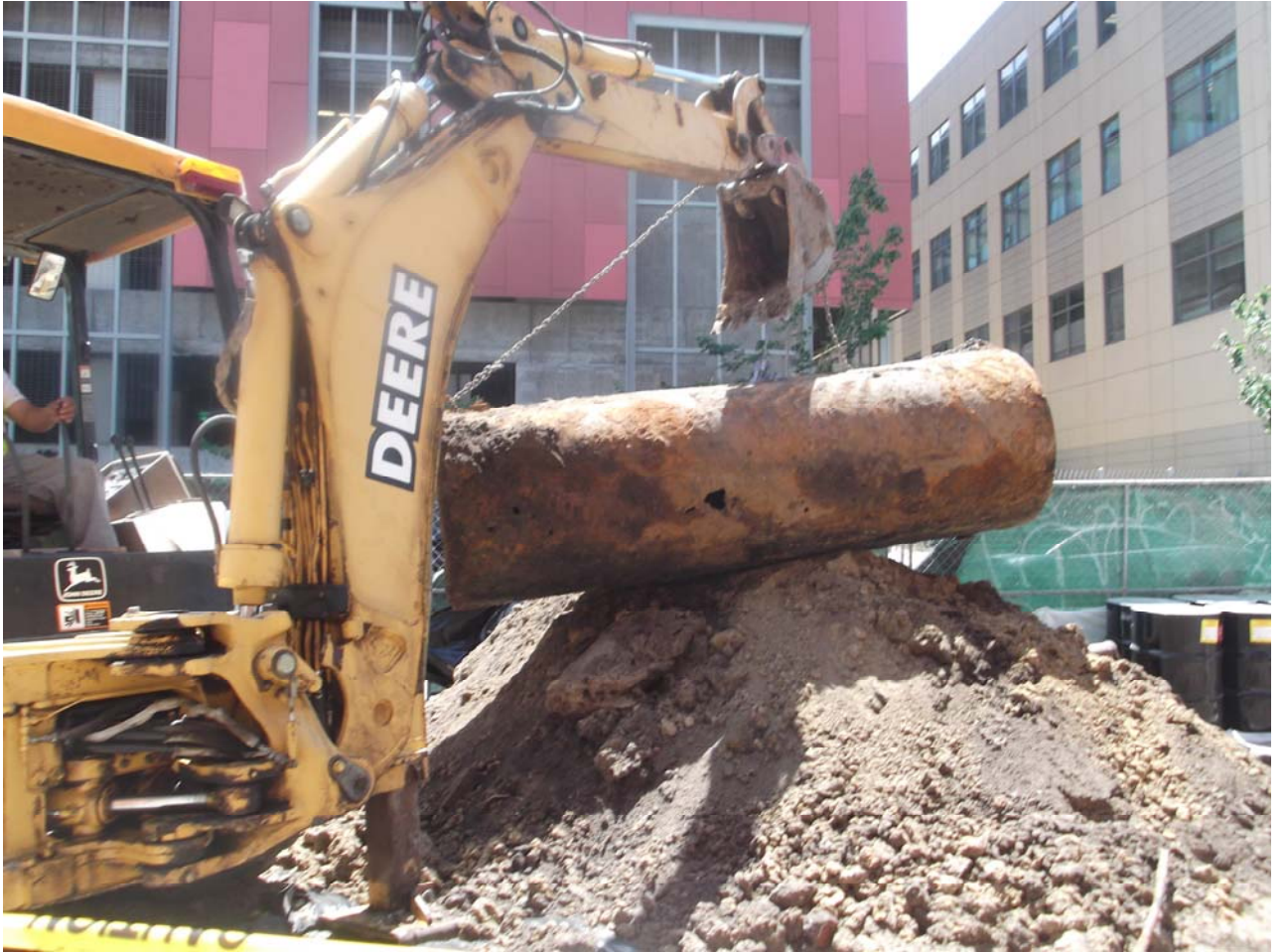
UST after removal
