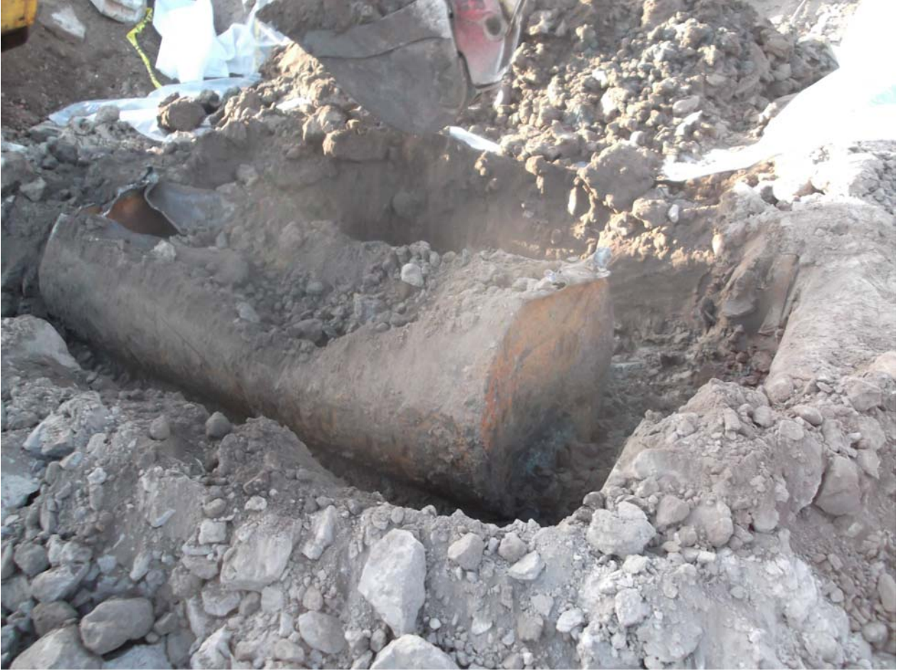
UST prior to removal
