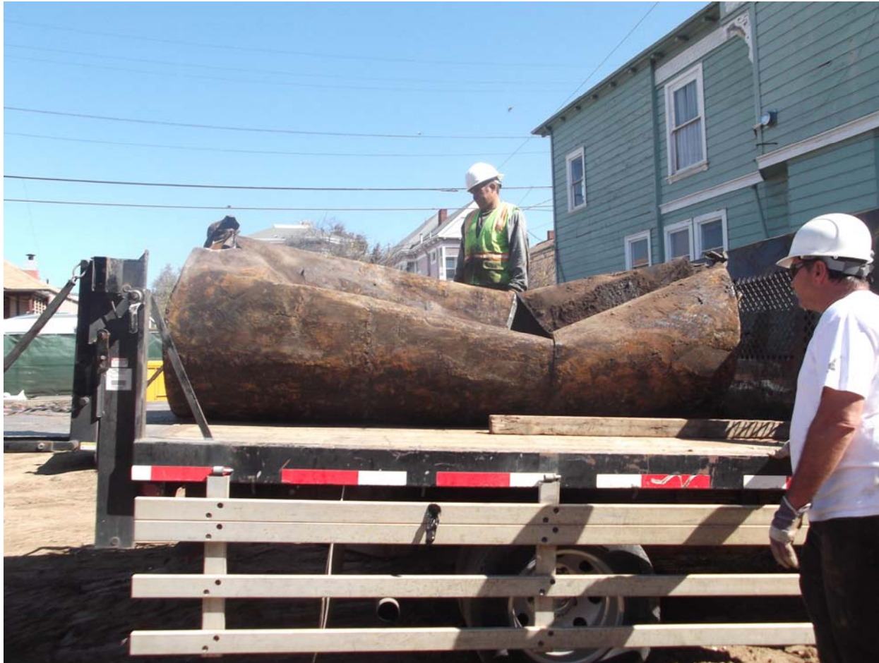
UST following removal
