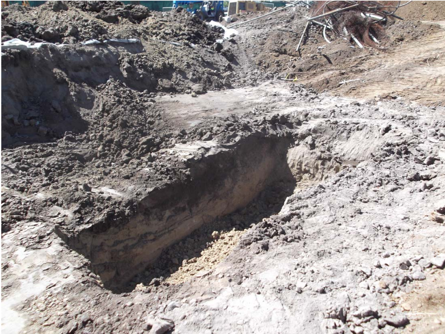
UST pit following tank removal
