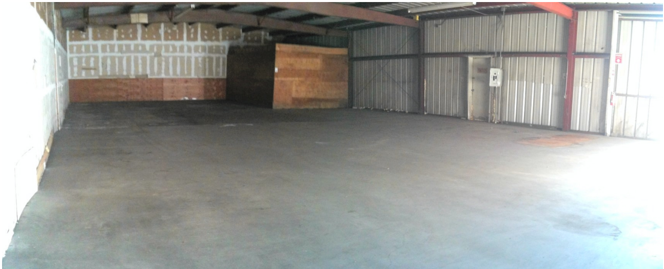
Photo 14: Subject Site (Facing East) Building 4 (Dry Goods Storage Building) Former Dry Goods Storage Warehouse
