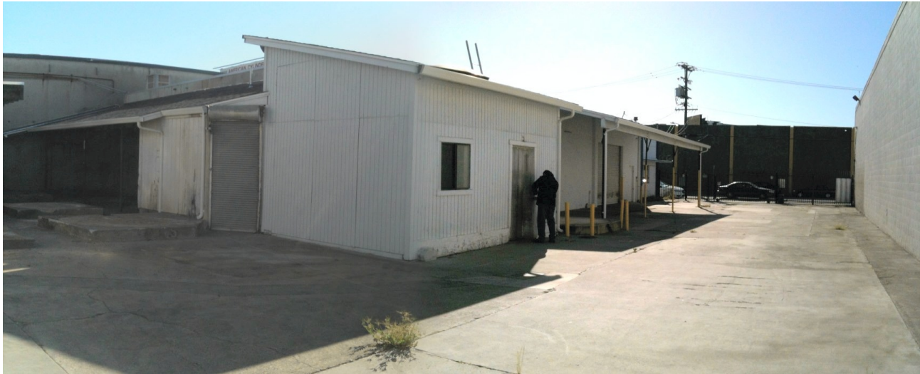
Photo 4: Subject Site (Facing Southeast) Building 1 (Office/Processing Area) and Associated Paved Areas
