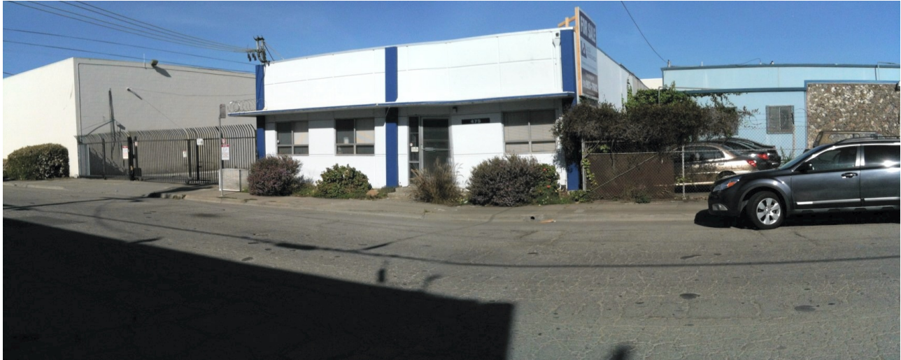
Photo 1: Subject Site (Facing Northwest) One-Story Commercial Office/Warehouse Buildings and Associated Paved and Landscaped Areas Along Northwest side of Lesser Street
