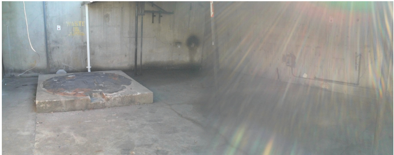
Photo 10: Subject Site (Facing East) Former Service Area Between Building 1 and Building 2 Concrete Pads for Former Sugar/Syrup ASTs, Boiler and Air Compressor
