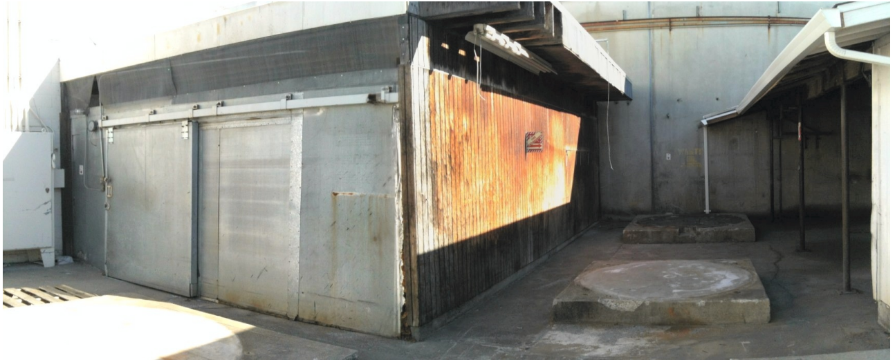
Photo 8: Subject Site (Facing North) Building 2 (Cold Storage Shed)
