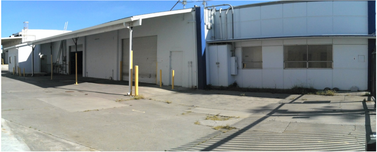
Photo 3: Subject Site (Facing Northeast) Building 1 (Office/Processing Area) and Associated Paved Areas
