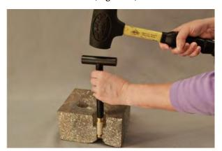
Figure 3. Flush-mount installation.
