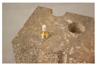
Figure 4. Installed Vapor Pin<sup>TM</sup>.
