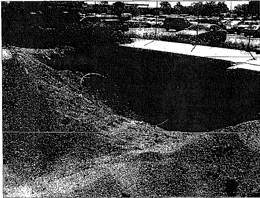
Open excavation pit following UST removal
