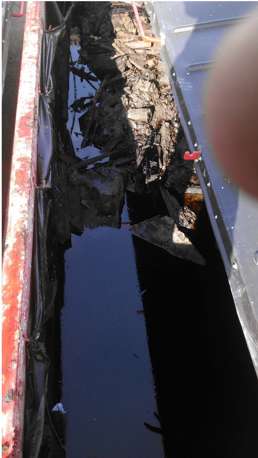
Photo 7. Soil and Debris Disposed as Non-RCRA Hazardous Waste
