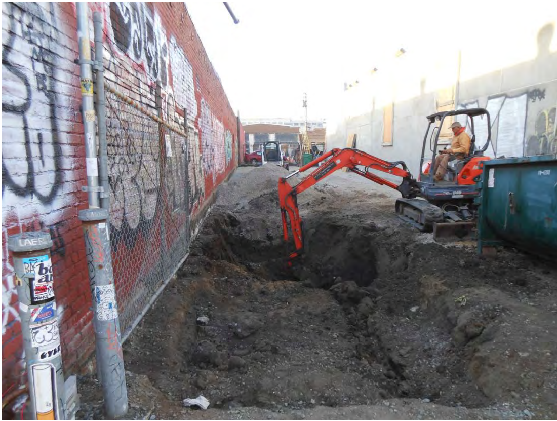
Photo 5 Proximity of UST Excavation to Adjacent Building
