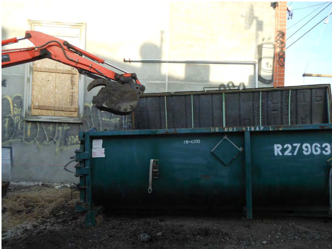
Photo 4 Loading Contaminated Soil into Roll-Off Bin
