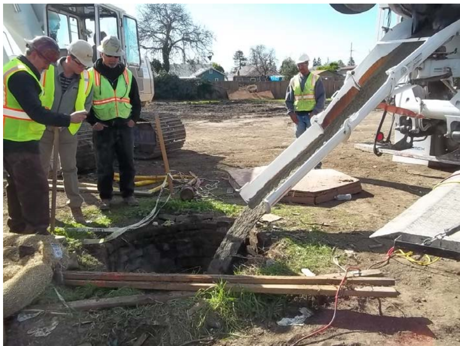
Photograph 4: Backfilling the water cistern with cement grout.
