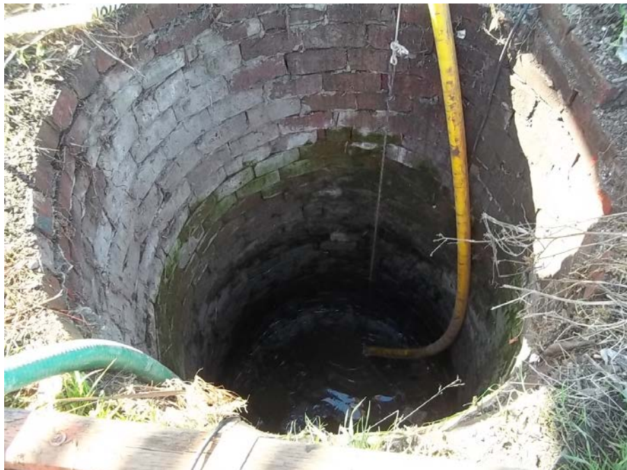
Photograph 2: Pumping water from water cistern.
