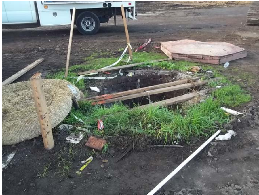
Photograph 1: The water cistern prior to abandonment activities.
