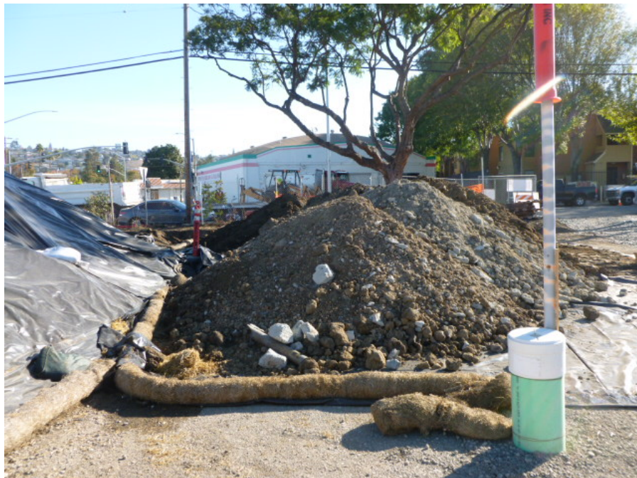
Photograph 16: Stockpiles SPB and SPC generated from trenching in Kent Avenue.
