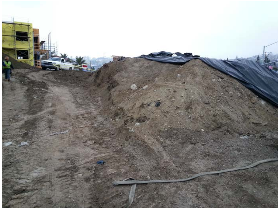
Photograph 18: Stockpile SPE generated from soil excavated from the Building A footprint.
