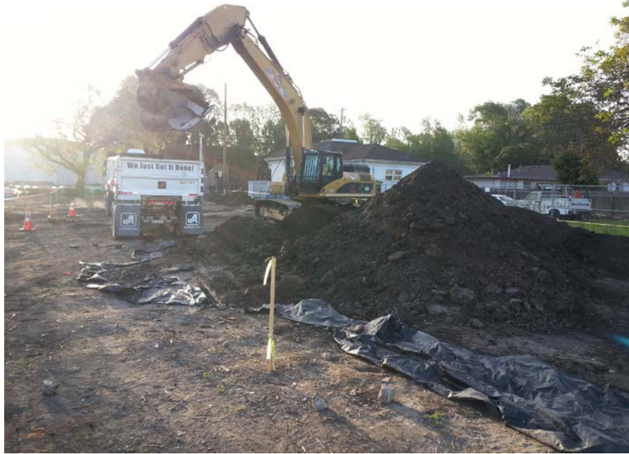
Photograph 13: Loading stockpile SP8 on to trucks for off-site disposal.
