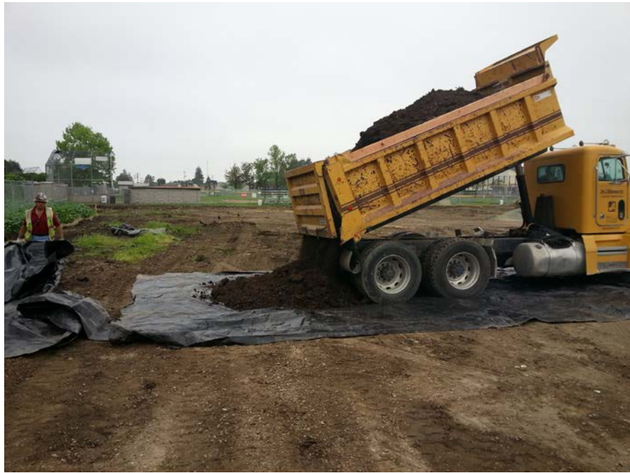
Photograph 7: Generating stockpile SP8 from the remedial excavations.
