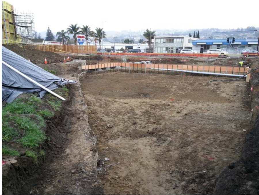
Photograph 17: Excavation in the Building A footprint to pour cellcrete.
