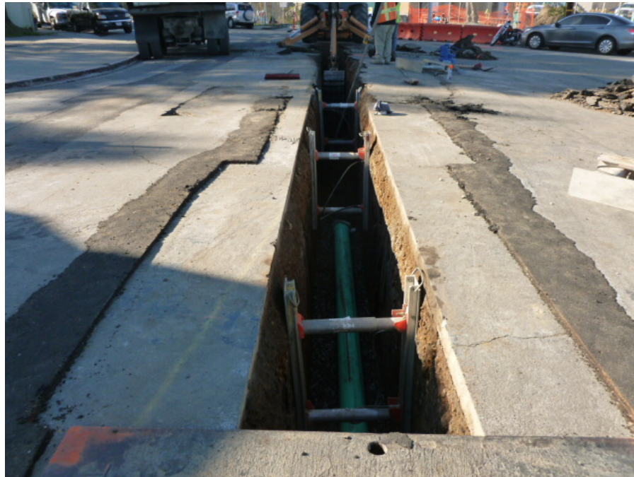
Photograph 15: Trenching in Kent Avenue.
