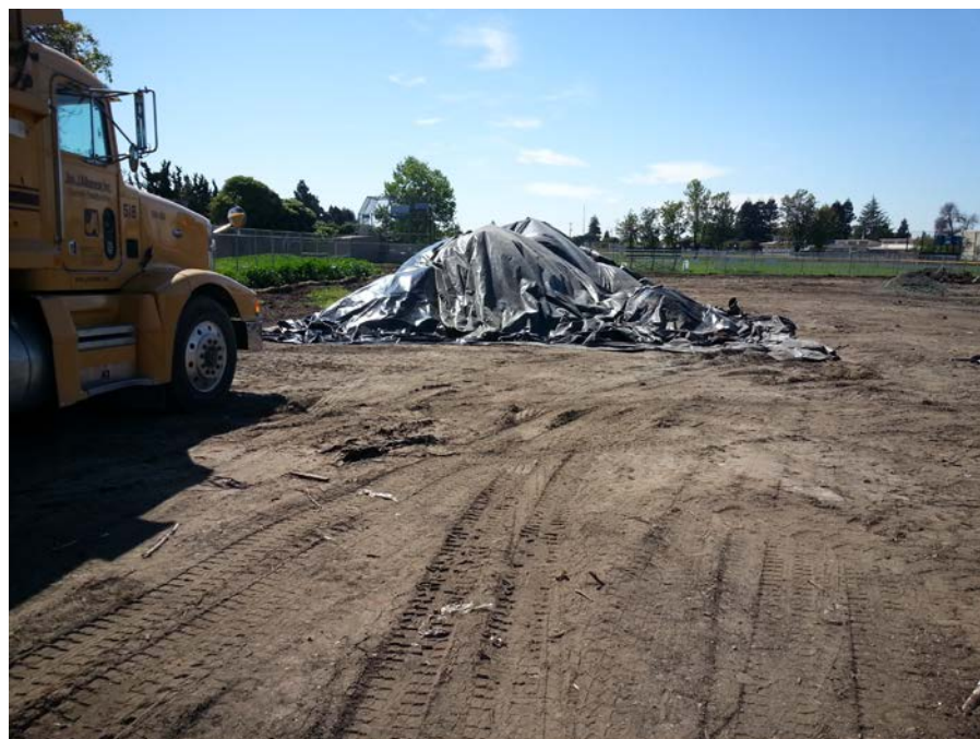
Photograph 12: Stockpile SP8 generated from remedial excavation of impacted soil.
