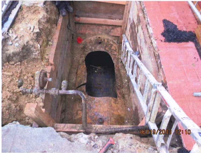
UST READY TO BE REMOVED FROM EXCAVATION
