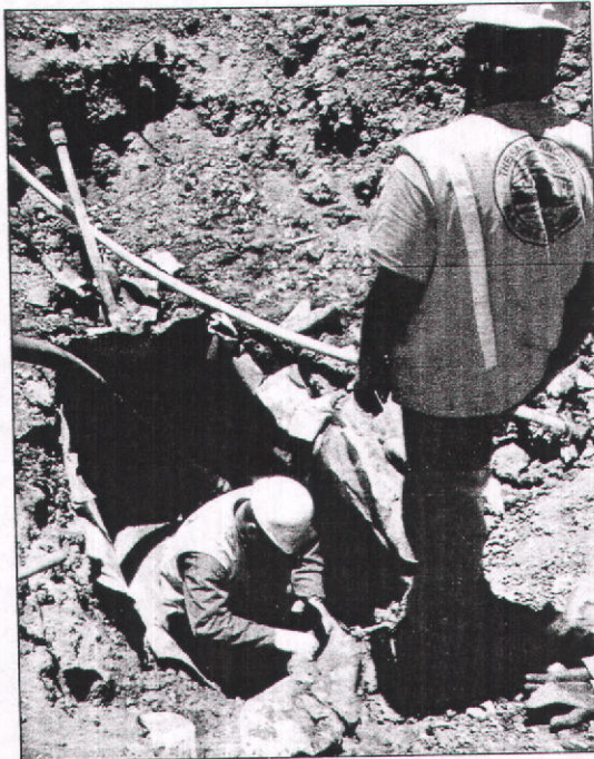
UST IN EXCAVATION BEING READY FOR REMOVAL
