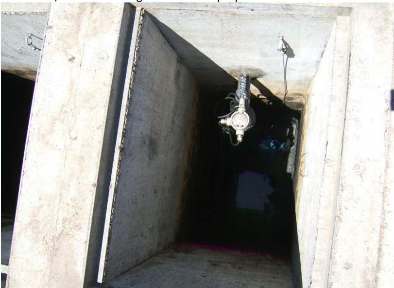
3. June 23, 2010 – View from about a vault sump.
