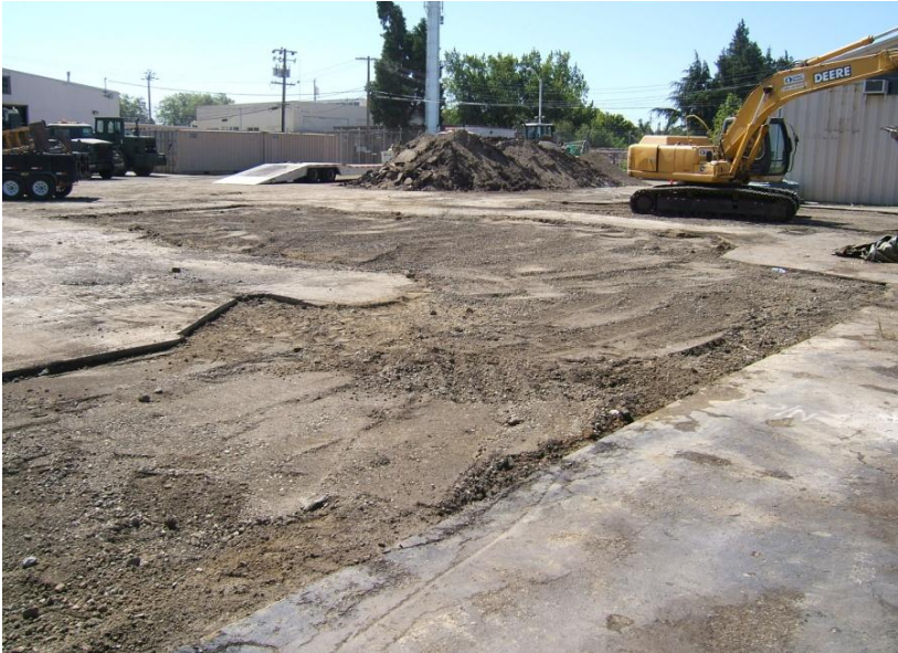
17. June 30, 2010 – Preparation of excavation areas prior to asphalt application.
