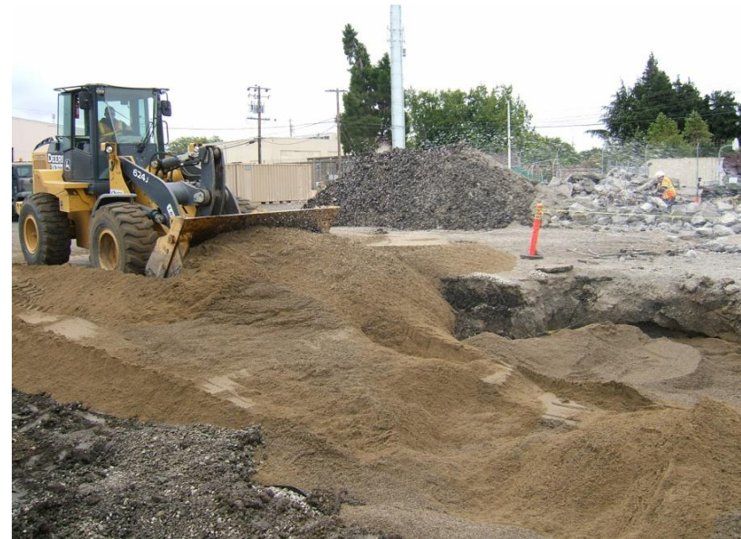
14. June 25, 2010 – Spreading of sand over geotextile fabric.
