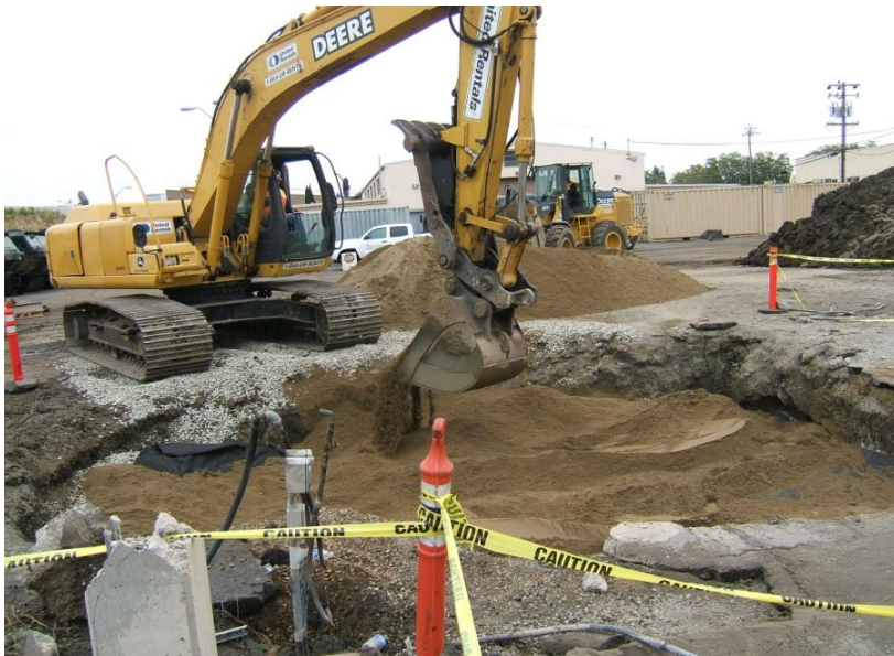
13. June 25, 2010 – Sand placed over drainage rock and geotextile fabric.
