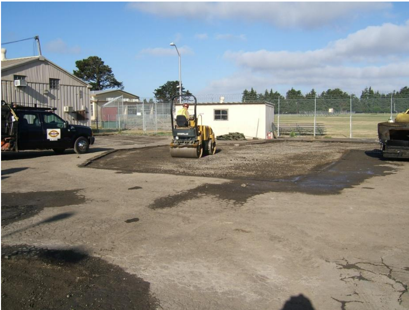
21. July 1, 2010 – Compacting the base prior to asphalt application.
