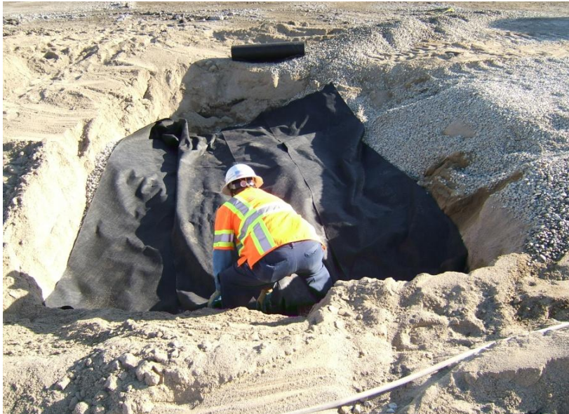
15. June 28, 2010 – Insertion of geotextile fabric over drainage rock.
