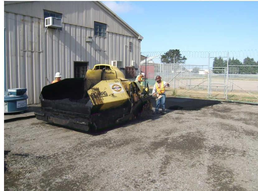
22. July 1, 2010 – Start of asphalt application near maintenance building.
