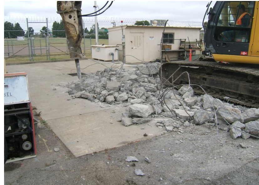
8. June 24, 2010 – Demolition of the concrete prior to the removal of rebar.
