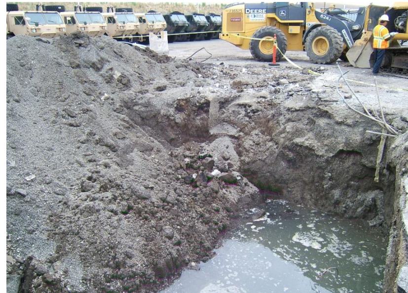
6. June 24, 2010 – Groundwater present within the excavation.
