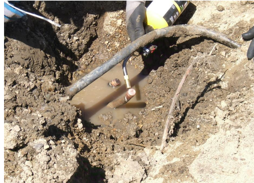
16. June 28, 2010 – Cut and capping of piping.
