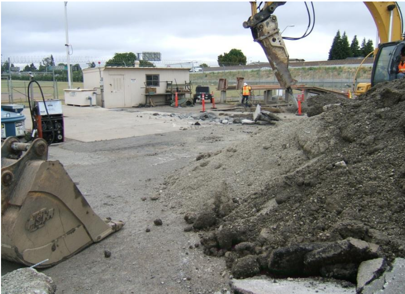
7. June 24, 2010 – Further concrete removal around sump vaults.
