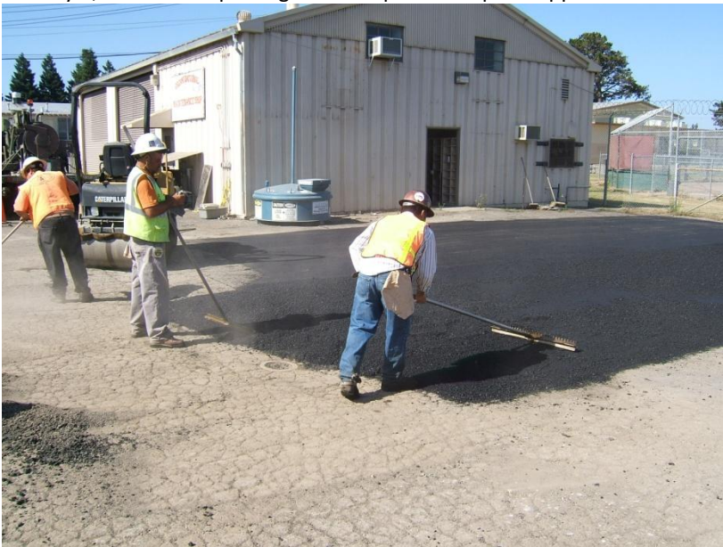
23. July 1, 2010 – Spreading of asphalt to match surrounding area.
