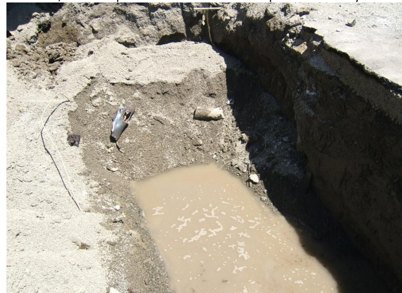
4. June 23, 2010 – Groundwater was reached during excavation activities.
