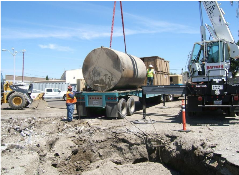
5. June 23, 2010 – Removal of the UST and transportation via flat-bed truck.
