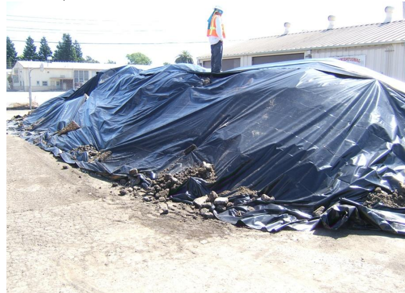
20. June 30, 2010 – Protection of stockpiled soil with high-density polyethylene prior to removal.
