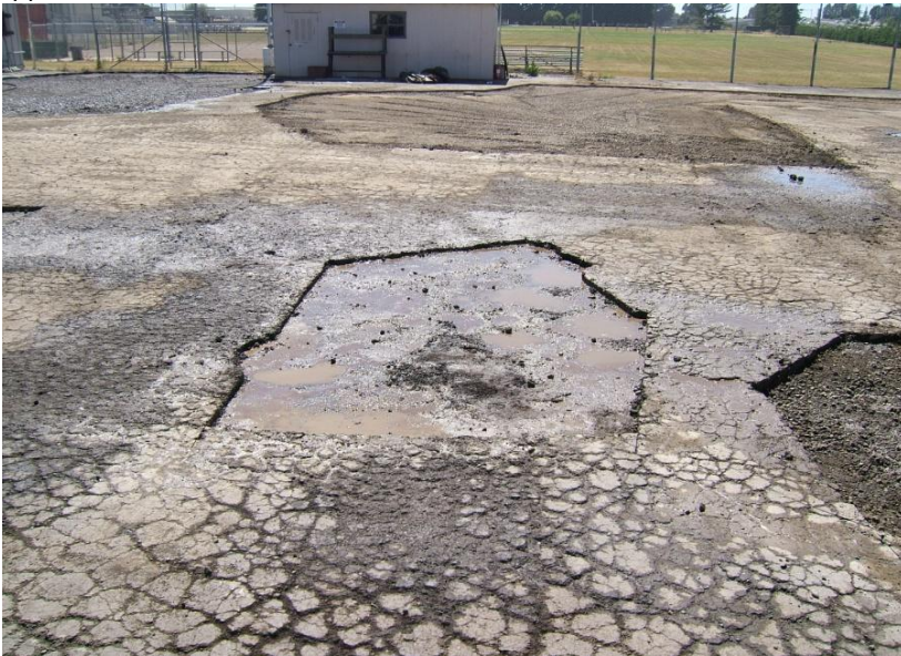
19. June 30, 2010 – Excavation areas prepared for arrival of asphalt.
