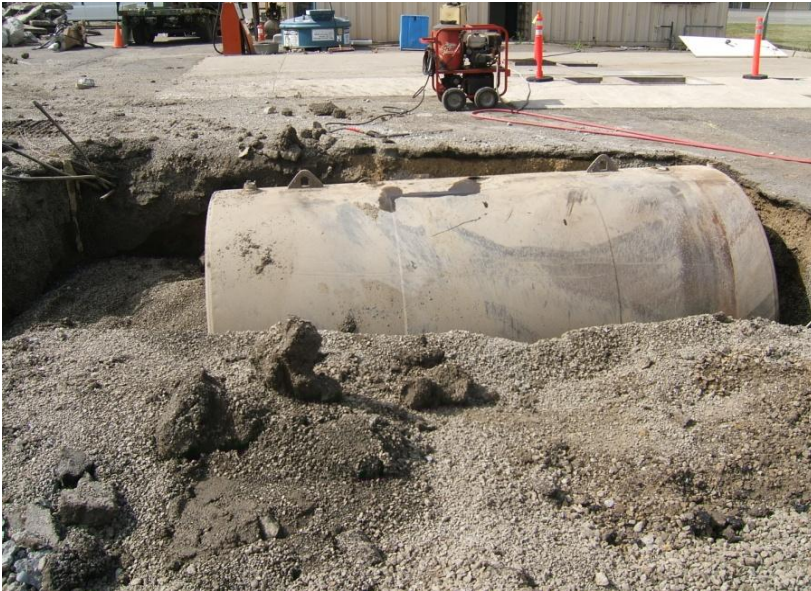
1. June 23, 2010 – Clearing of the UST to prepare for removal.
