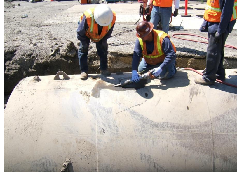
2. June 23, 2010 – Expansion of vent to allow the placement of dry ice.
