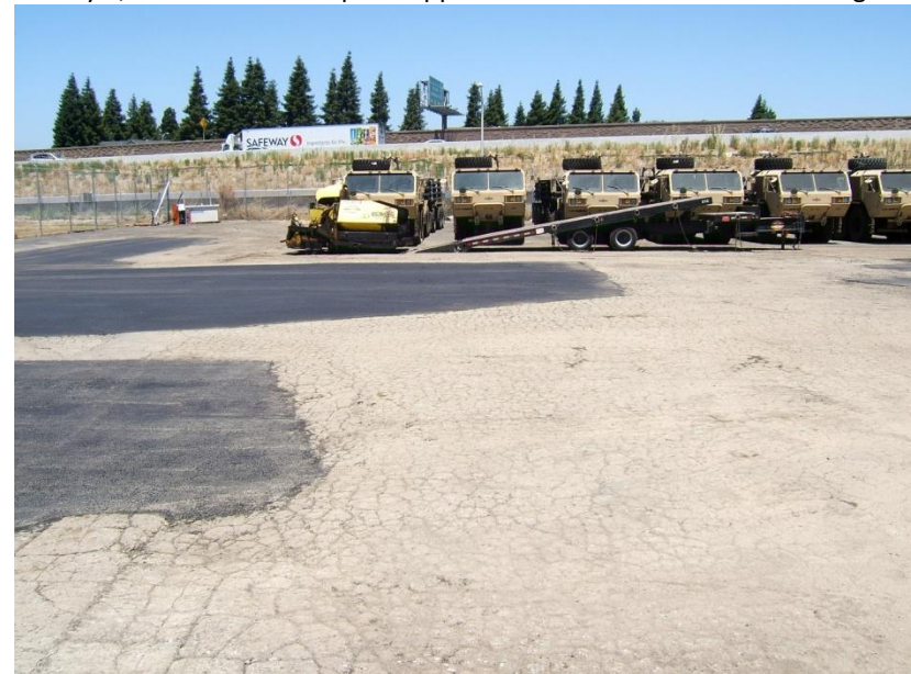
24. July 1, 2010 – Finished asphalt at the San Lorenzo yard.
