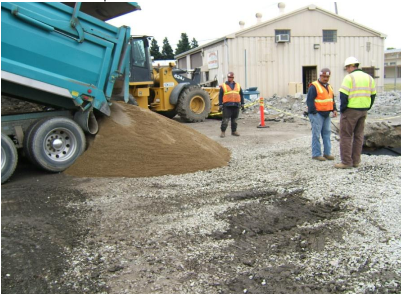
11. June 25, 2010 – The arrival of sand to be placed within the excavations.
