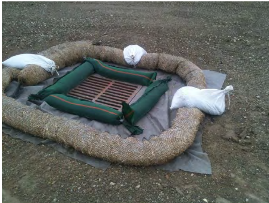
Photo 4: Storm drain on Site
