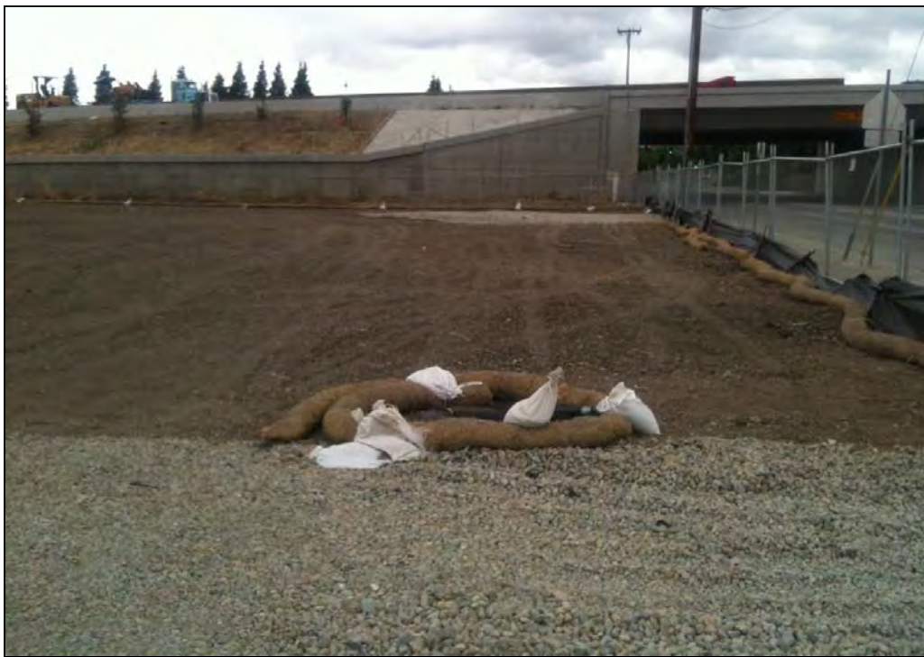
Photo 2: View of the Site.
