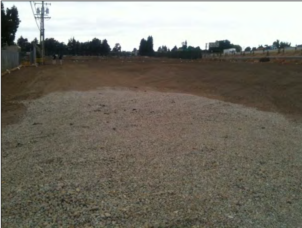
Photo 1: View of the Site
