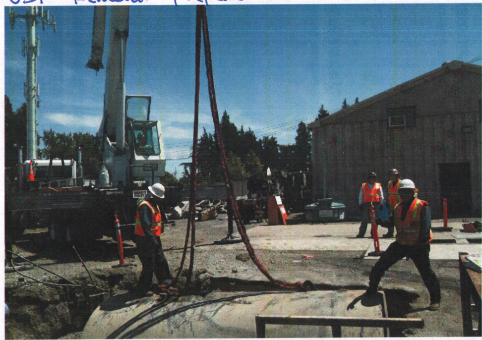
UST Removal preparation
