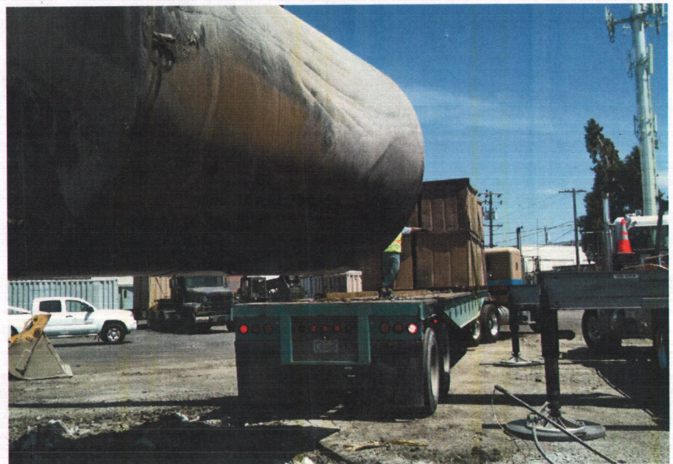
UST Removal and loading
