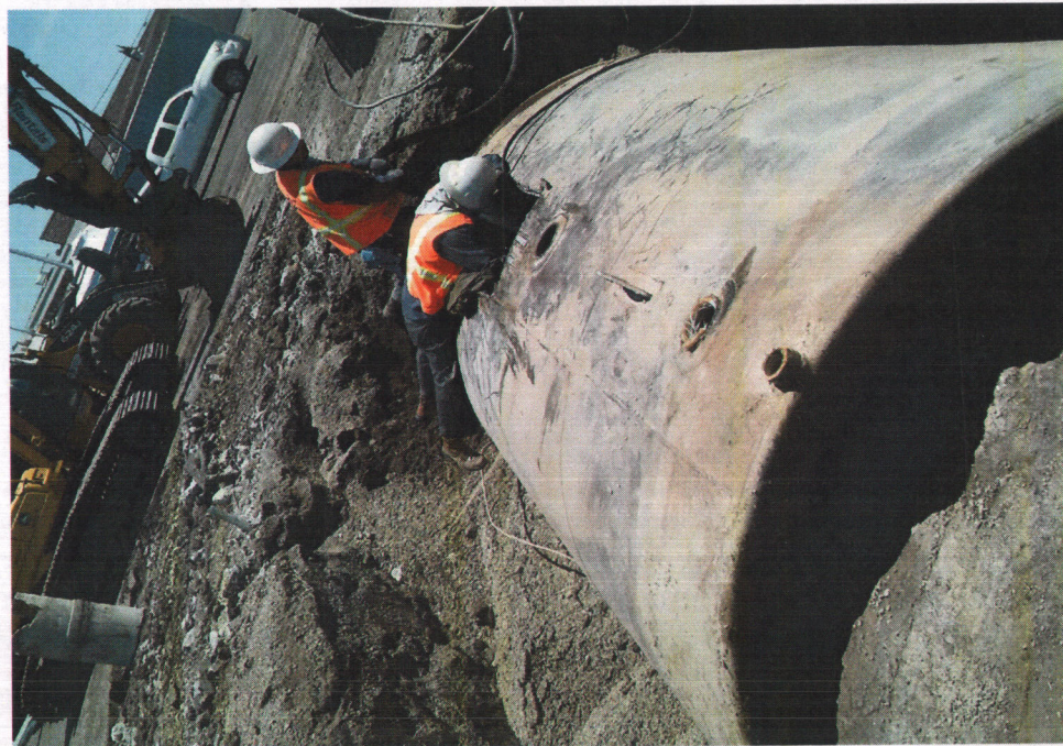
UST prep for removal
