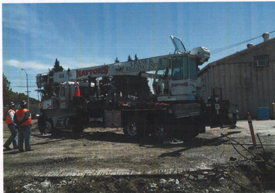
Crane for UST removal
