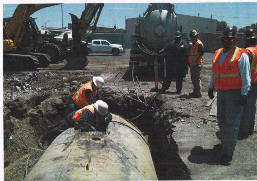
UST Removal preparation
