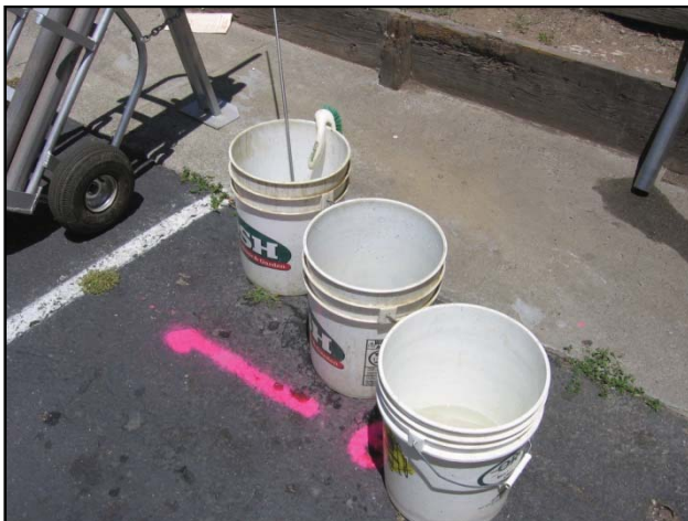
Photograph 5: Drill rods were decontaminated in between borings to prevent cross contamination.
