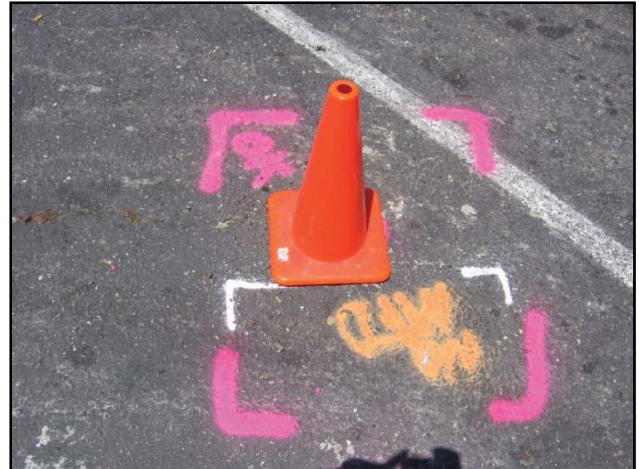
Photograph 2: Prior to drilling, boring locations were cleared for subsurface utility lines.
