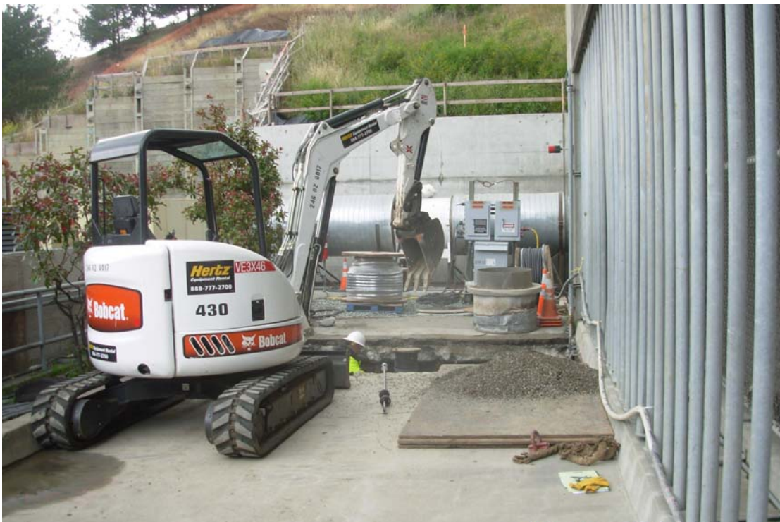
Photo 4 – View of mini excavator used to remove pea gravel from excavation.
