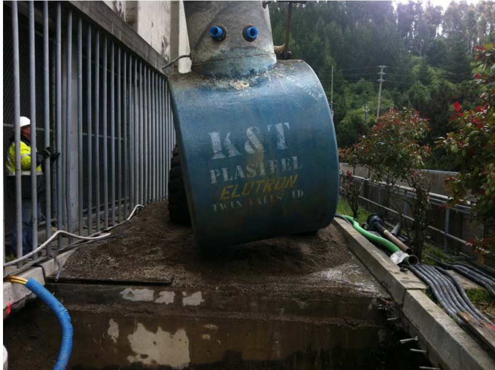
Photo 5 – View of UST being hoisted from the excavation by loader.
