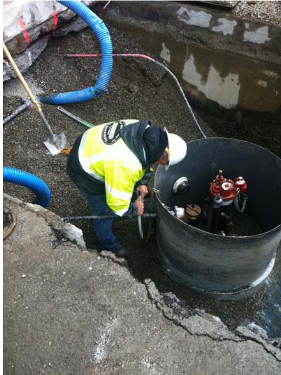
Photo 3 – View of electric and fuel lines being disconnected from UST.
