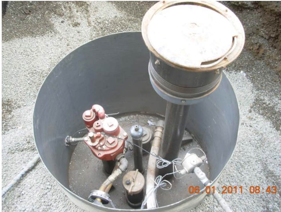
Photo 1 – View of appurtenances located on top of UST prior to removal.
