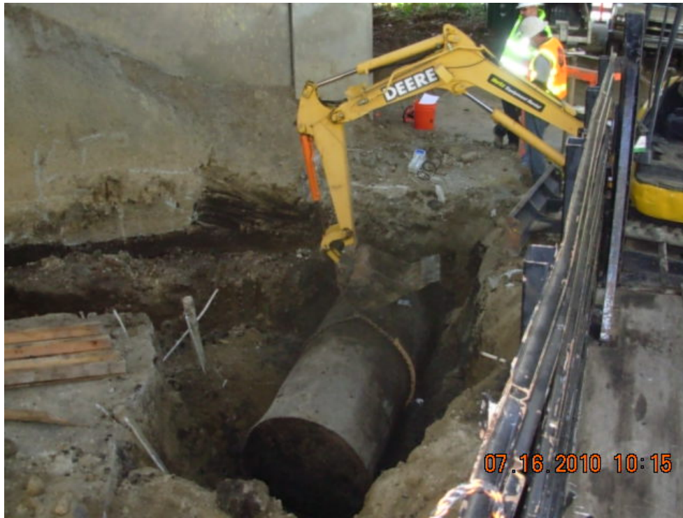
Photograph 5 – View of UST being removed from the ground.
