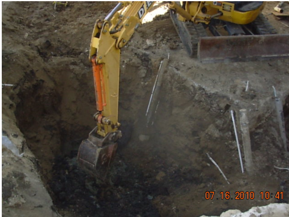
Photograph 4 – View of excavation and surrounding soil nails
