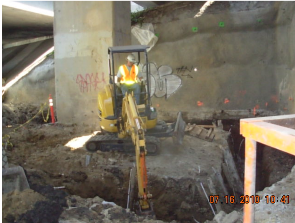
Photograph 3 – View looking east at UST excavation and immediate surrounding area.
