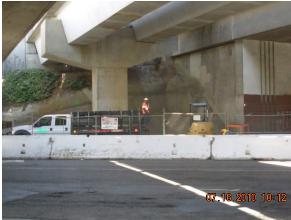
Photograph 1 – View looking east across Telegraph Avenue at UST removal area.
