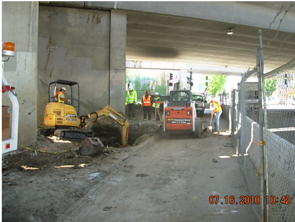
Photograph 2 – View looking south at UST removal area.
