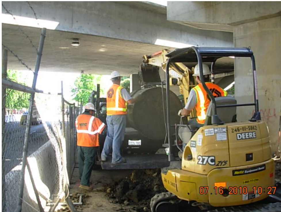
Photograph 6 – View of UST being loaded onto NRC truck for disposal.
