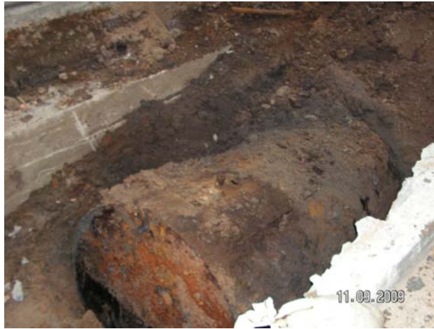
Photo 4 – View of top of UST after it had been unearthed.
