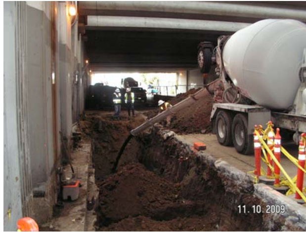
Photo 7 – View of excavation being backfilled with sand slurry on 10/10/09.
