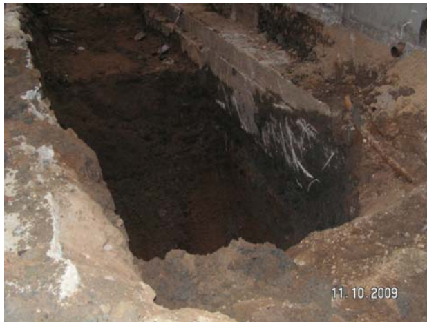
Photo 6 – View of tank pit after over excavation on 10/10/09.
