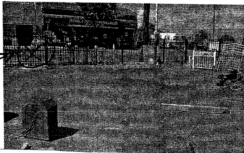
. A picture of a suspected UST location area on the subject property.
