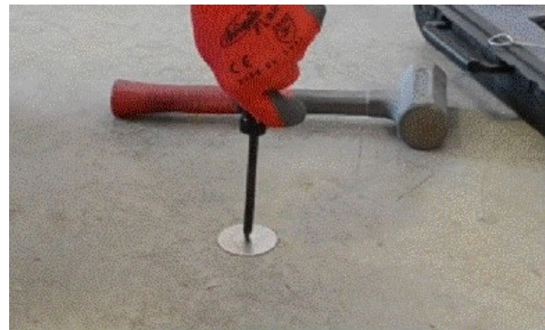
Figure 5. Tightening the Secured Cover.
